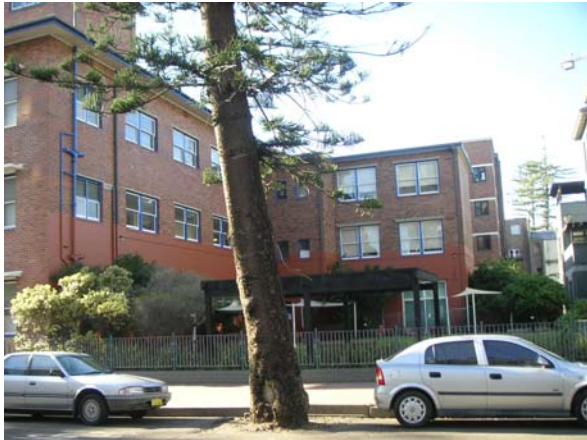
West elevation (left) and extension to Drummond House (rear right)
