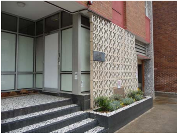
Main entry from Wentworth St
