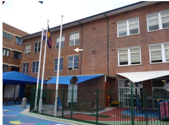
Southern addition indicated by different colour brick & arrow
