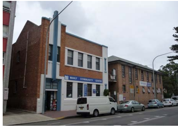
Manly Community Centre (left) and Manly Public School (right), 2011 (both heritage items)
