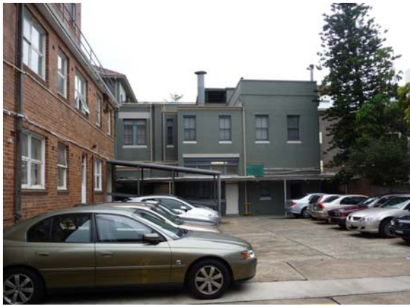
Western elevation of rear 1960s addition to Drummond House and Elsie Hill building (left) with rear car park
