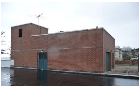
Figure 14 – Norman Drummond Building, external and internal spaces
