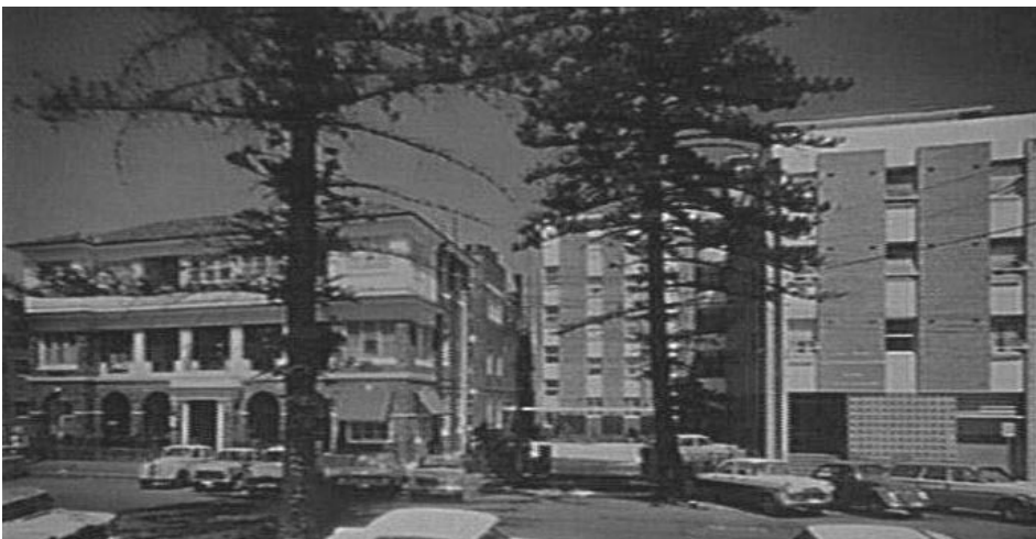
Figure 28 – Drummond House and Elsie Hill building on Wentworth St, c. 1962
