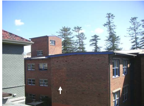
Rear of School; 1960 walkway link to Drummond House (left) demolished in early 1980s (indicated by arrow)
