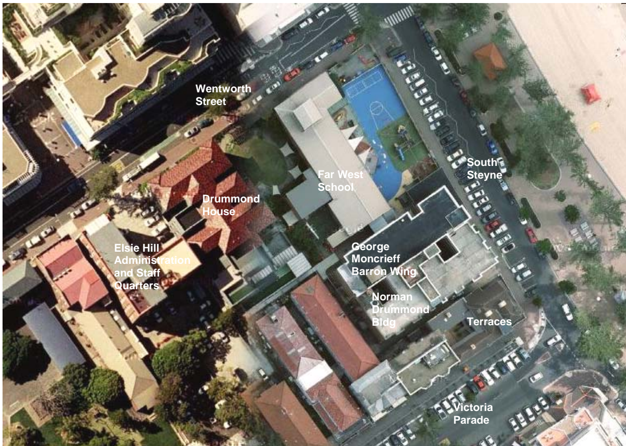
Figure 2 – Aerial view of site showing key buildings
