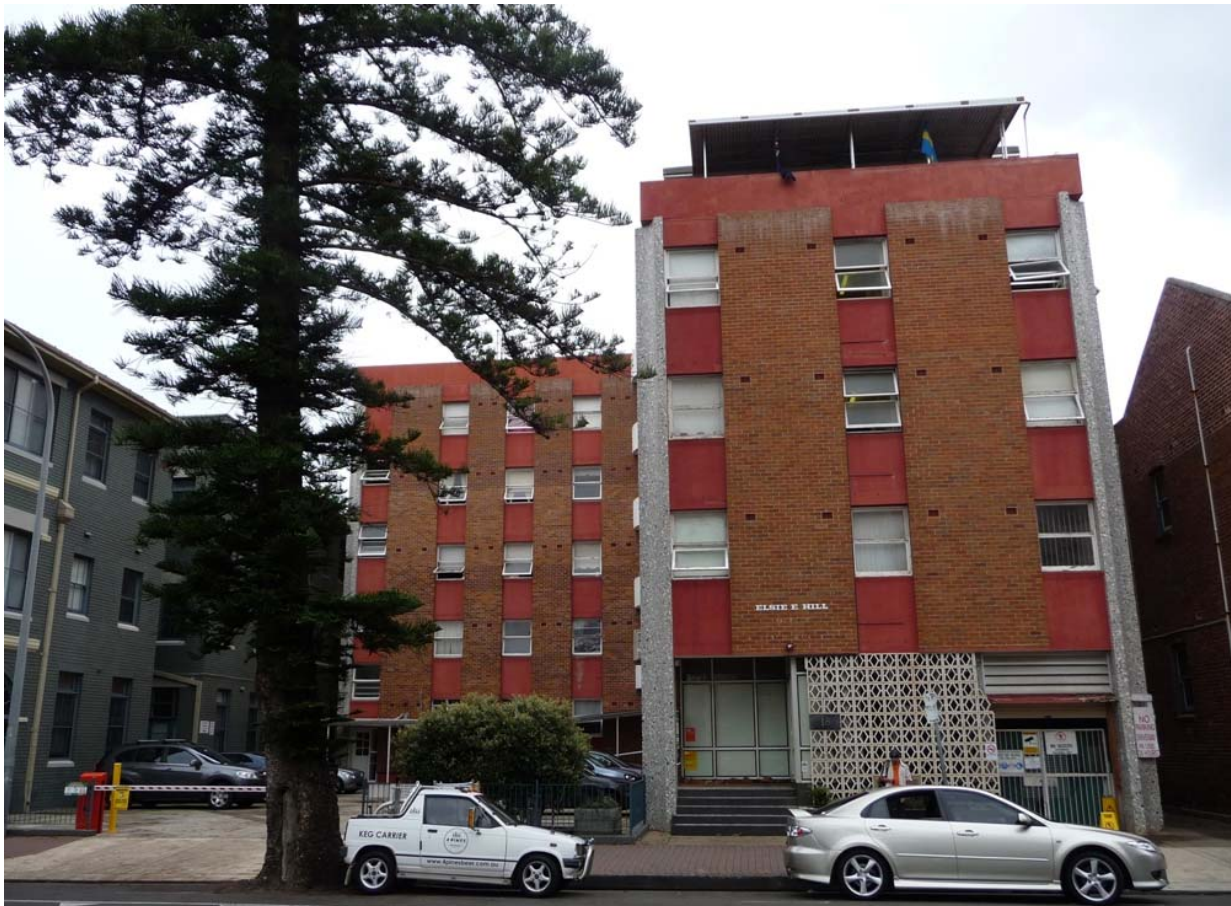
Figure 9 – Elsie Hill building
