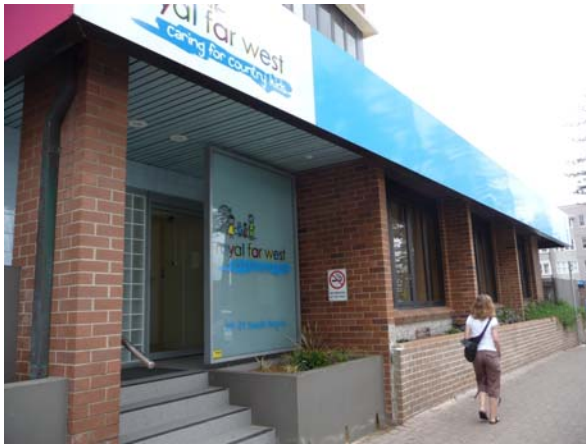
Detail of main elevation ground floor
