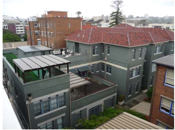
Roof and rear extension
