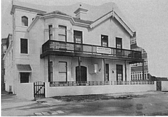
Figure 34 – House, No. 15 South Steyne, 1974 and 1986
