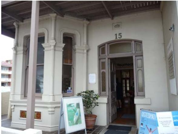
Ground floor, south section and main entry
