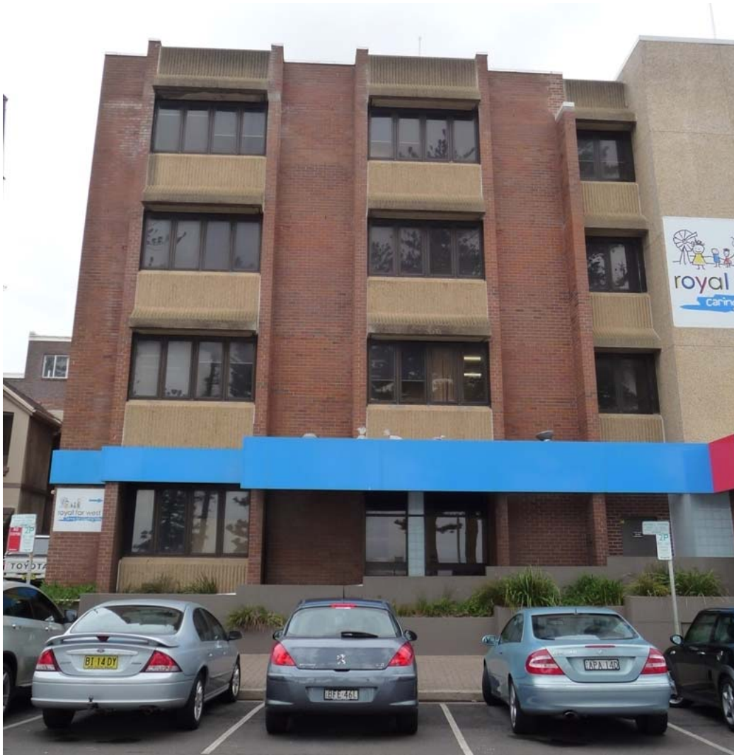
Figure 13 – Norman Drummond Building
