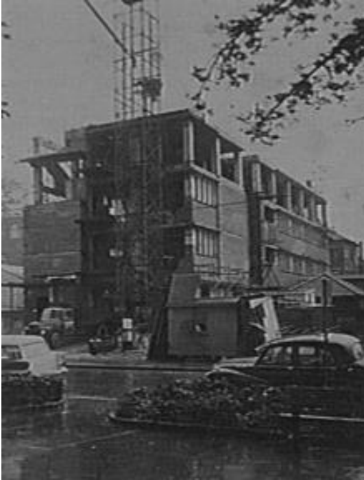
Figure 29 – Construction of the Moncrieff Barron Wing, 1964
