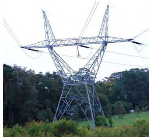
Figure ES-3 - H Steel Tower 330kV Tension Structure
