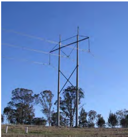
Figure ES-2 - H-Frame 330kV Supporting/ Intermediate Structure
