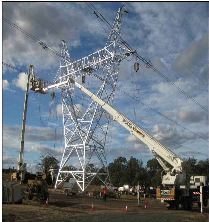
Plate 4-4 Termination Work Following Stringing
