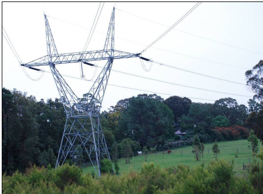
Plate 4-2 330kV Steel Tower Tension Structure
