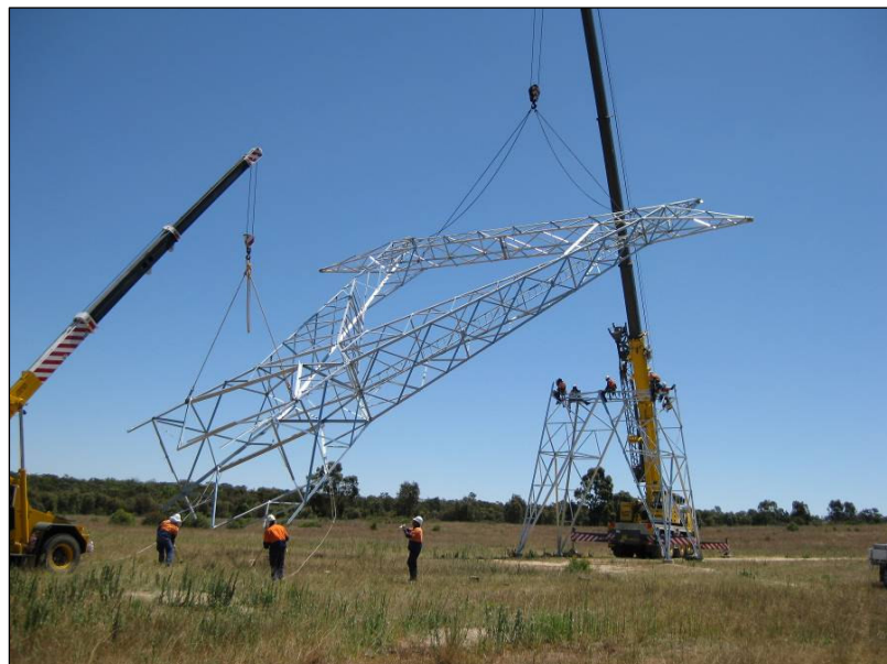
Plate 4-3 Steel Tower Assembly
