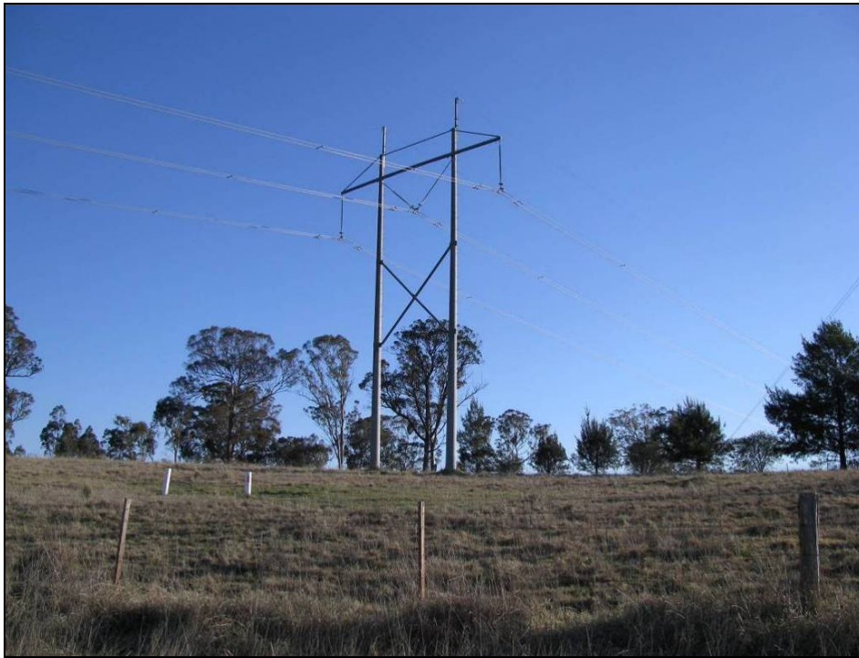
Plate 4-1 330kV H-Frame Supporting Structure
