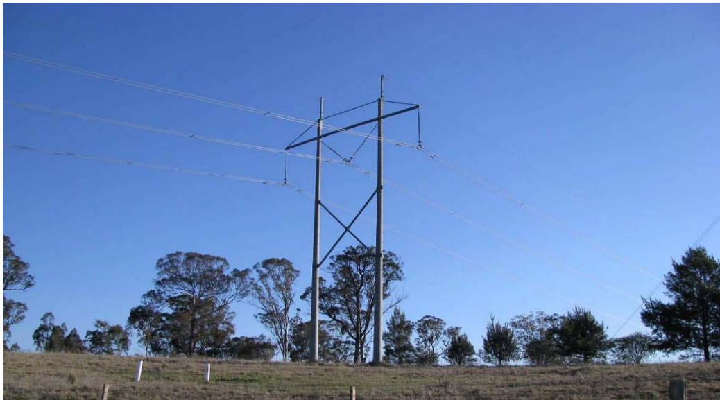
Plate 1-1 H-Frame 330kV Supporting/Intermediate Structure
