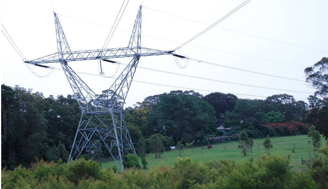
Plate 1-2 Steel Tower 330kV Tension Structure (Angle Position)
