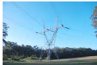
Plate 2 Indicative 330kV tension structure
