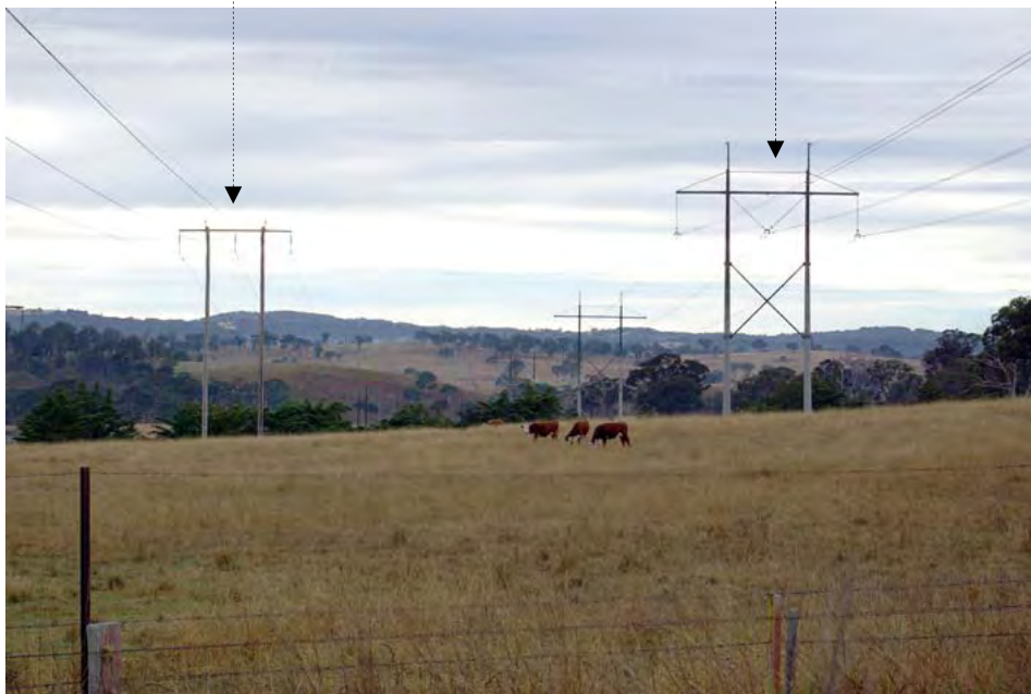
Plate 4. Existing 132kV twin pole transmission line and 330kV supporting structures north of the Armidale Substation.
