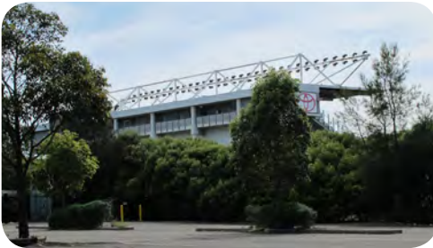
Carpark on western side of stadium
