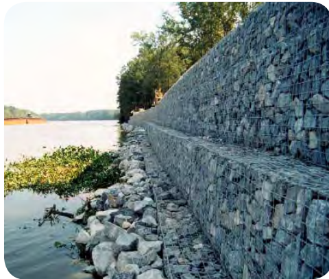
Bank stabilisation. Gabion walls > Georges River. ASPECT image library
