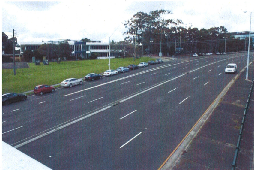
TUESDAY - north side Epping Rd from overpass
