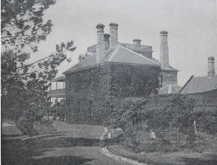
Figure 21 The east elevation of the house and the continuation of the brick-edged approach drive to the main yard to the rear in 1897. There appears to be a two-storey verandah on the west face of the kitchen wing. Note that the chimneys are of sandstone. Source: The Sydney Mail , 14 August 1897, pg 831.
