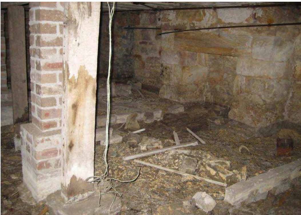
Figure 3.33 Basement room B3, showing masonry support for fireplace and additional brick pier and timber post supports. Source: Tanner Architects 2010.
