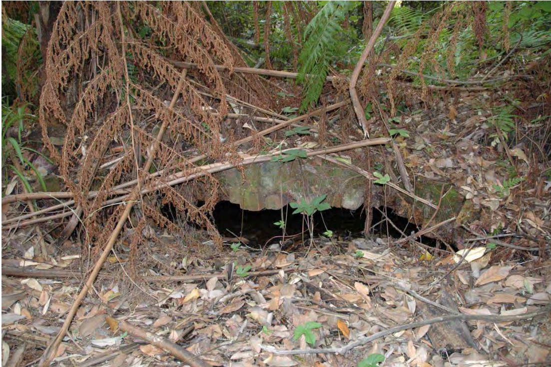
Figure 3.73 Photograph of the top of a brick arch—probably the roof of a brick cistern. The bricks are sandstock with a shallow 'cigar-shaped' frog. The bricks suggest a date of construction as no later than the 1860s. This cistern probably stored water to be used on the vineyard and orchard. Source: Mary Casey, 2010.
