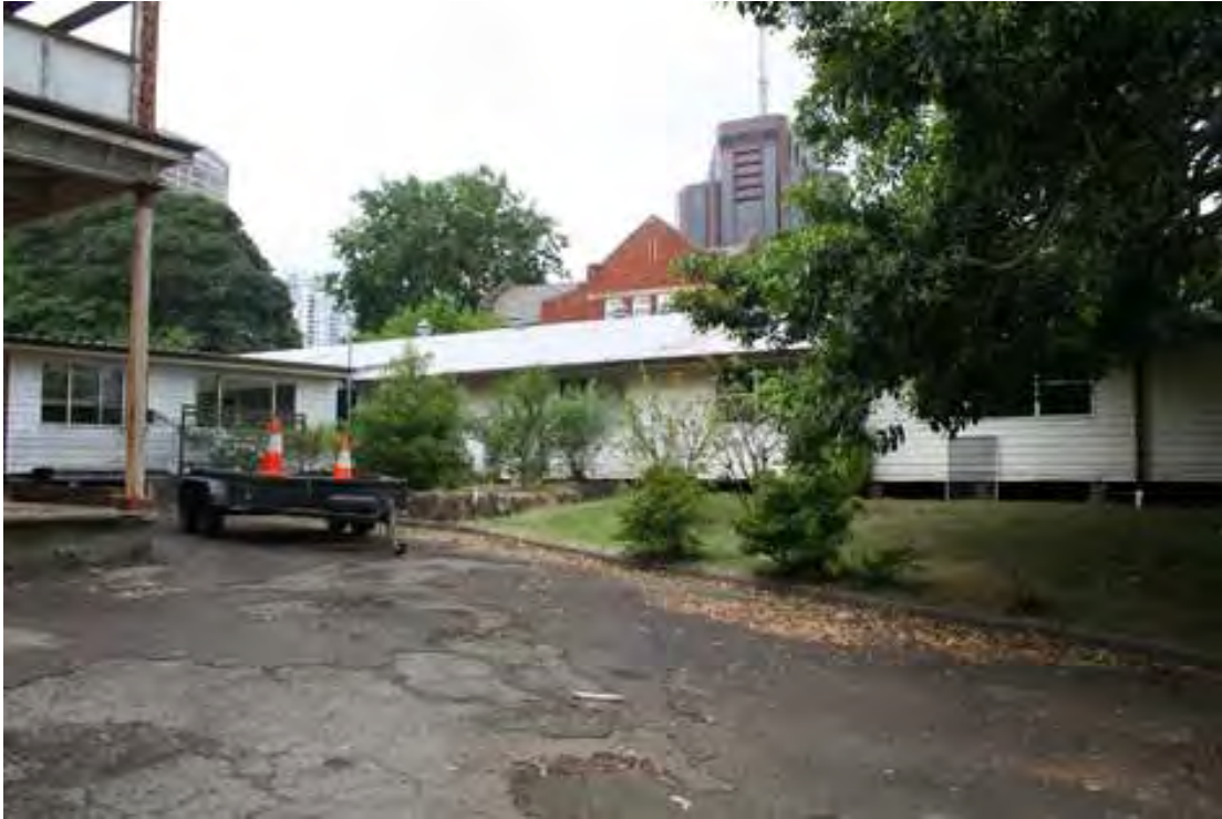
Figure 3.63 The west elevation of the Ward Building today. The original low-lying form of the building remains but the verandahs on both sides have been enclosed. Source: Tanner Architects 2010.
