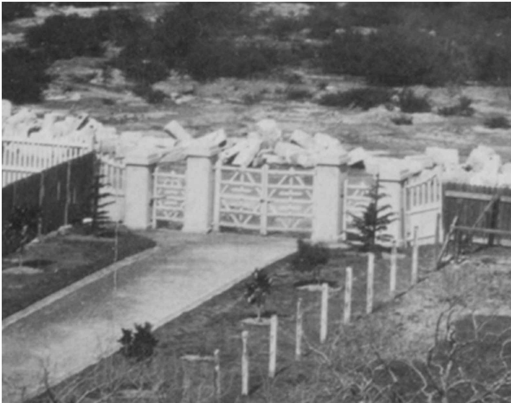
The Union Street entrance gates and driveway. Undated but possibly c1880. Source: National Library of Australia.
