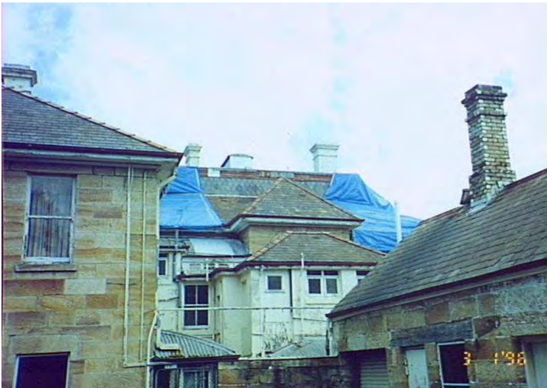
Figure 62 The rear elevation of the house in January 1996. The tarpaulins provide evidence of the damage to the roof caused by the collapse of two chimneys. They have since been rebuilt Source: Stanton Library Image 494.
