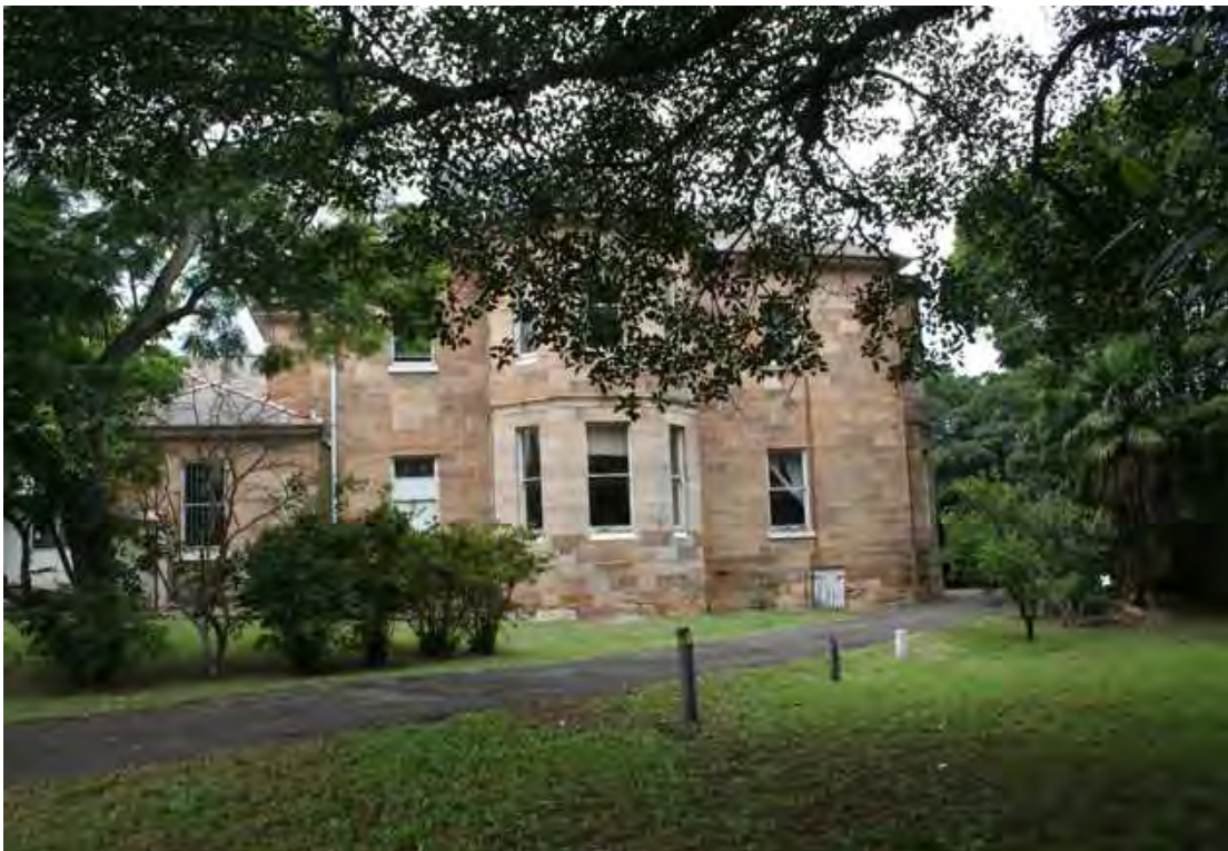
Figure 3.7 The west elevation of Euroka Villa (Graythwaite) today showing the 1870s remodelling by George Dibbs including the removal of the upper level balcony and the construction of the bay windows. Source: Tanner Architects 2010.
