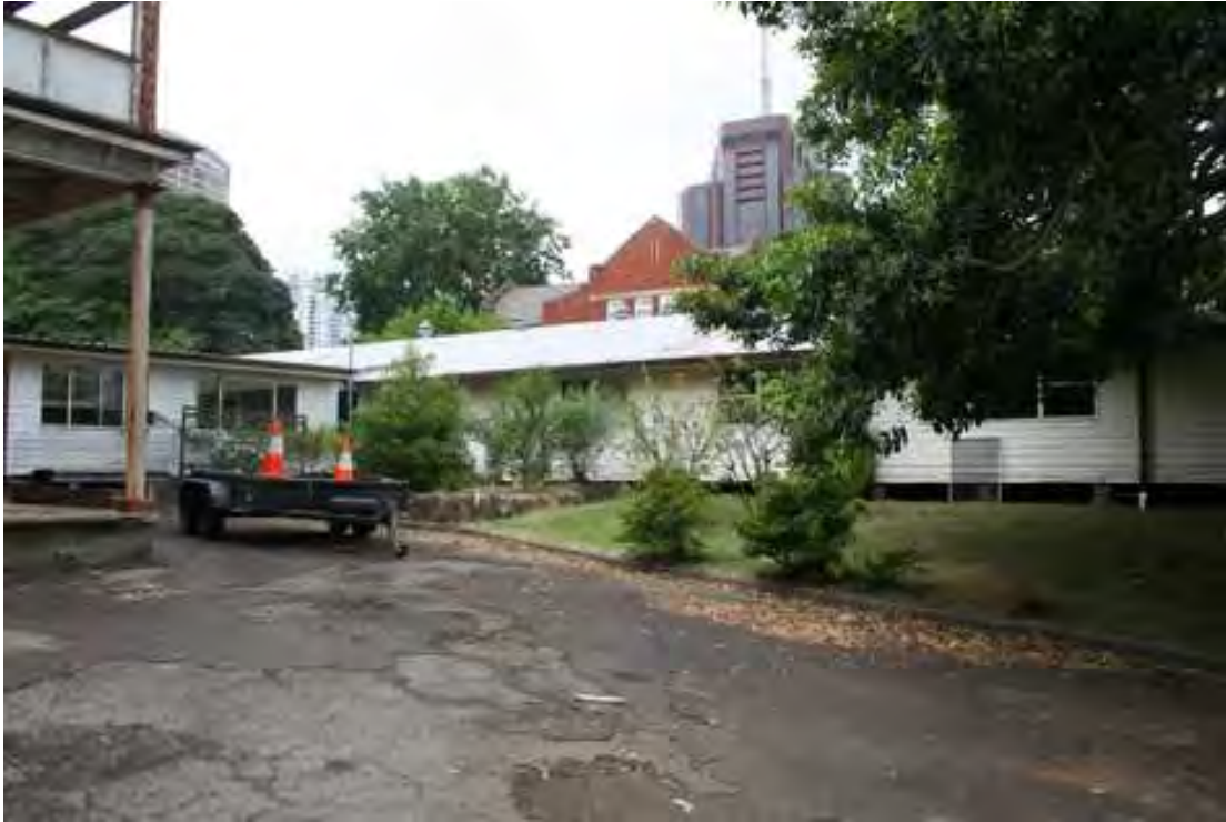
Figure 3.41 The west elevation of the Ward Building today. The original low-lying form of the building remains but the verandahs on both sides have been enclosed. Source: Tanner Architects 2010.
