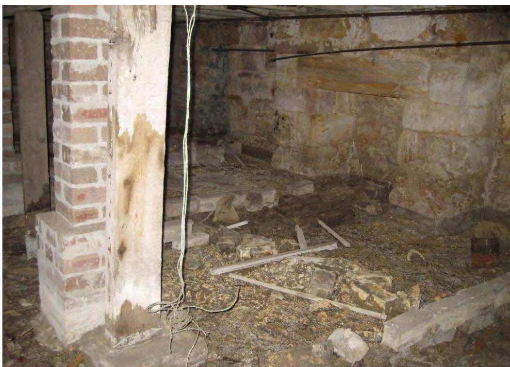
Figure 3.22 Basement room B3, showing masonry support for fireplace and additional brick pier and timber post supports. Source: Tanner Architects 2010.
