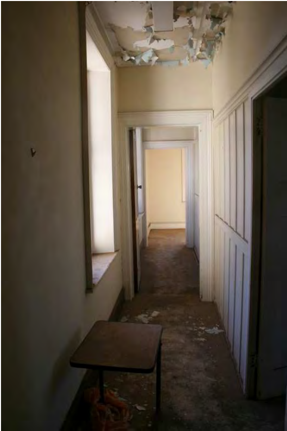
Room F10A. Looking north. The 1924 timber partitions and mid-twentieth century upper level infill are at right.
