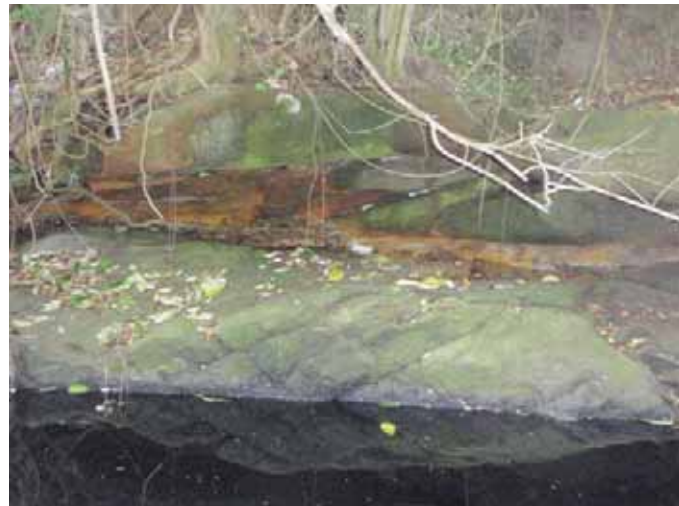
Sandstone walls of stormwater drainage canal
