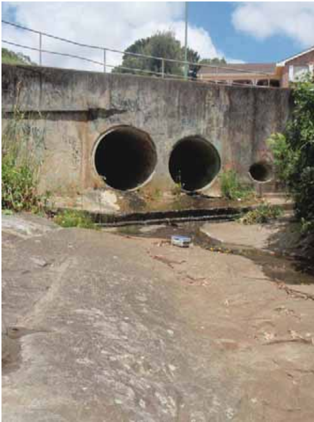
View of stormwater outlet pipes beneath Stirling Avenue
