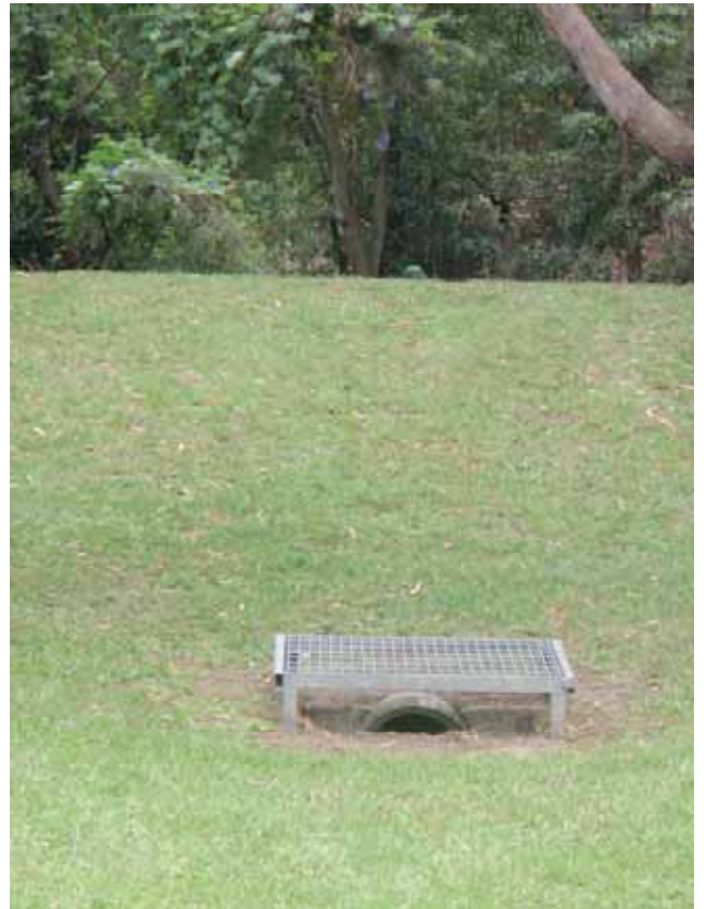
Above: inlet to stormwater pipe at down gradient section of park
