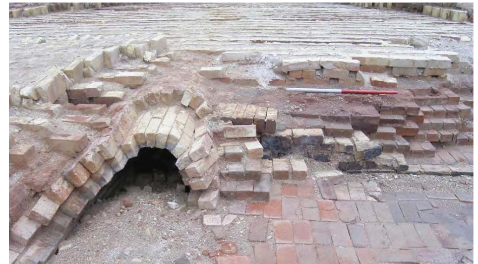
Photograph of Kiln 1 showing the layer of flues and floor (courtesy of Edward Higginbotham & Assoc).
