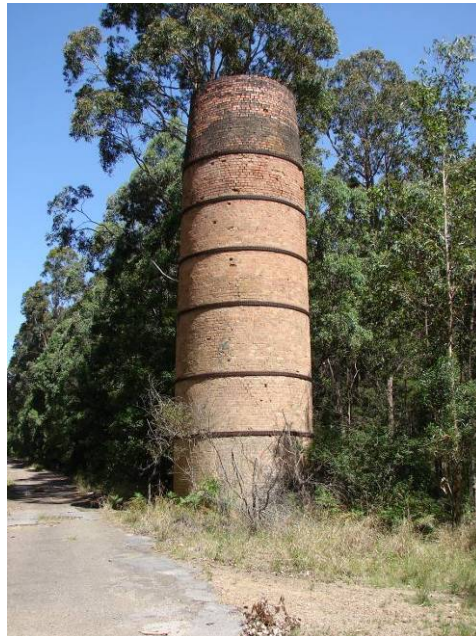
Photograph 5.25 Air Furnace Shaft Duckenfield No 2 (ERM 2007)
