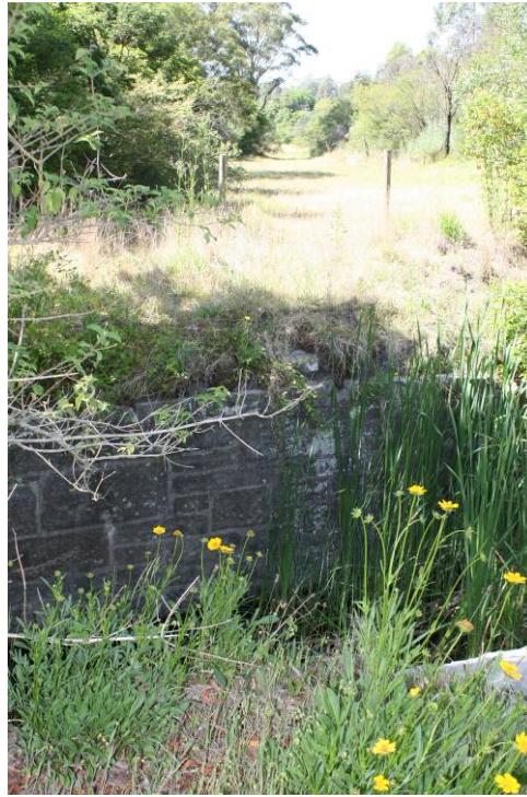
Photograph 5.6 View south east over Minmi Creek showing bridge abutments and railway alignment along the valley floor (ERM 2007)
