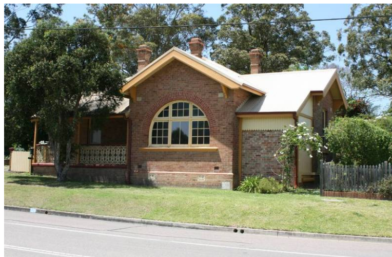
Photograph 5.12 Former Minmi Post Office and Residence view form the west (ERM 2007)
