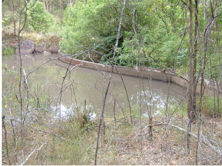
Photograph 5.40 Wall of the brick dam
