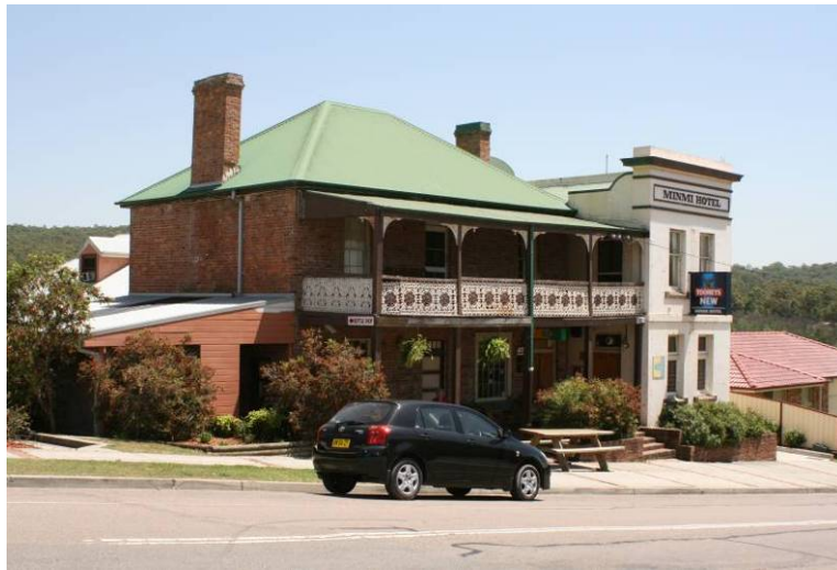
Photograph 5.9 Minmi Hotel from south east (ERM 2007)
