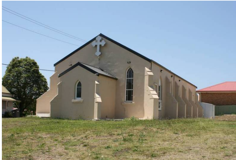
Photograph 5.16 View from Church Street (ERM 2007)
