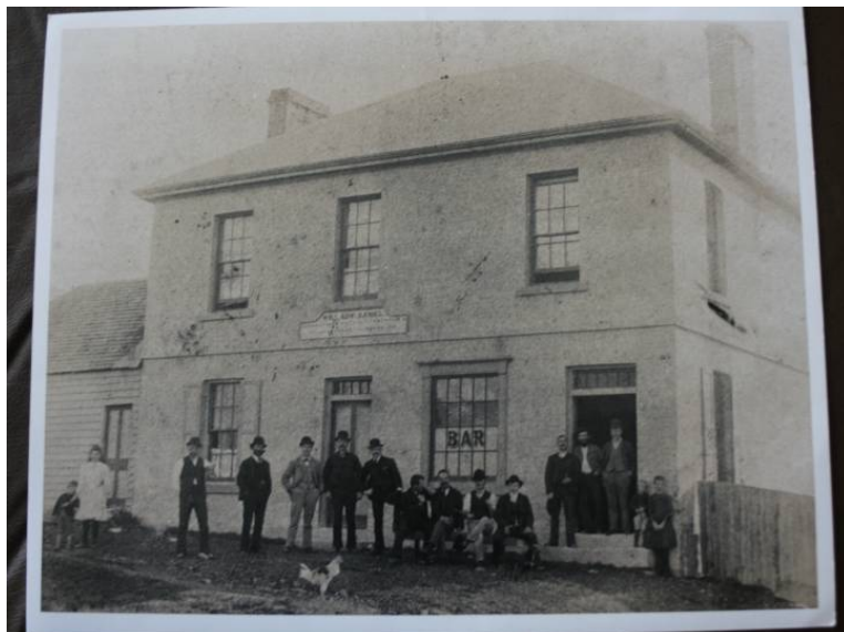
Photograph 5.10 Minmi Hotel from south east (from personal collection of Kerry Hinds)
