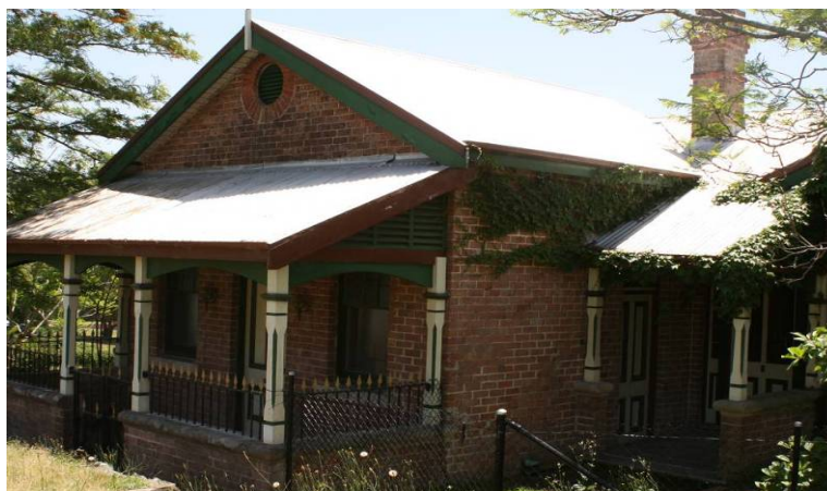
Photograph 5.14 Court House viewed from the south east.
