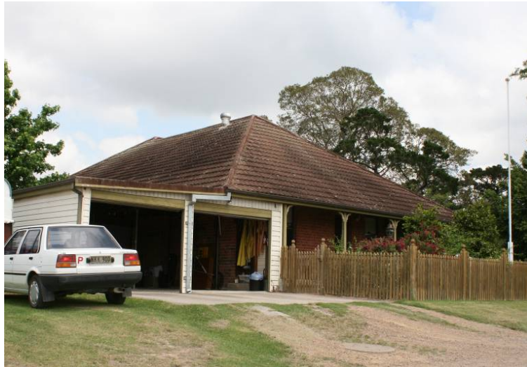
Photograph 5.1 Former Minmi Reservoir Residence. View from north east (ERM 2007)Former Minmi Public School, 196 Woodford Street
