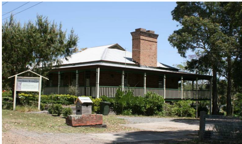
Photograph 5.13 Police Station viewed from the north east.
