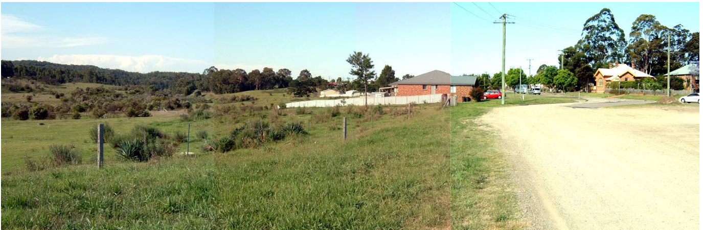
Photograph E.3 Photograph montage to coke oven site, facing N. Railway Street is the road on the right. Post Office can be seen on right centre. Ambulance Station stood where red brick house now is.
