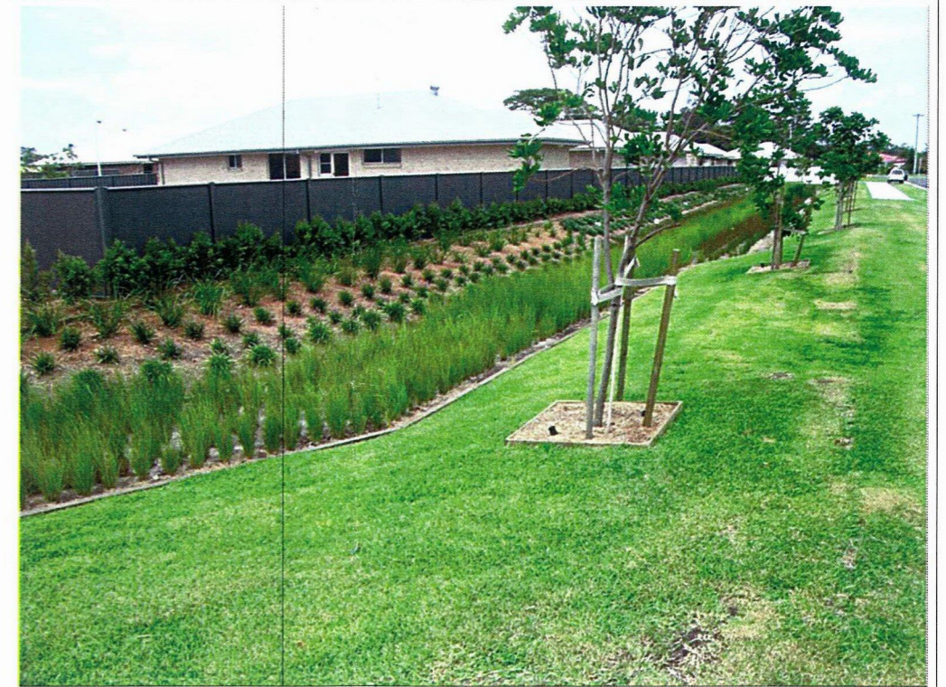
PHOTO 1: EXAMPLE OF RECENTLY CONSTRUCTED BIOFILTRATION BASIN WITH A WIDTH OF APPROXIMATELY 4m
