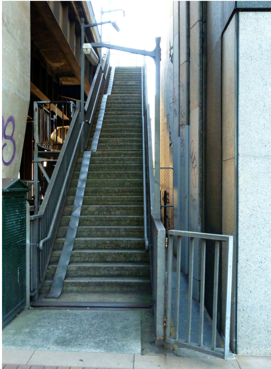
Figure 10 – Stair between Macquarie Street and the Cahill Expressway
