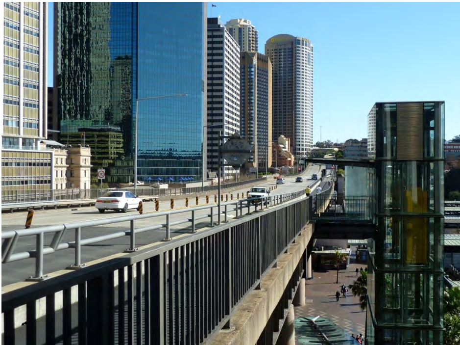
Figure 12 – The Cahill Expressway looking west
