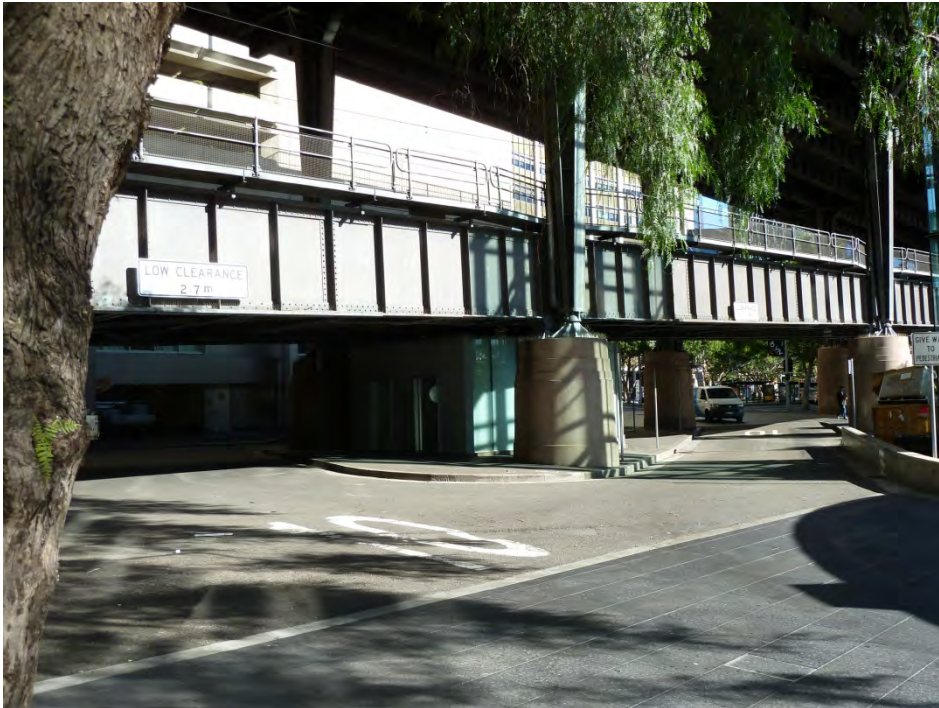
Figure 14 – Access road with restricted height clearance under the rail viaduct
