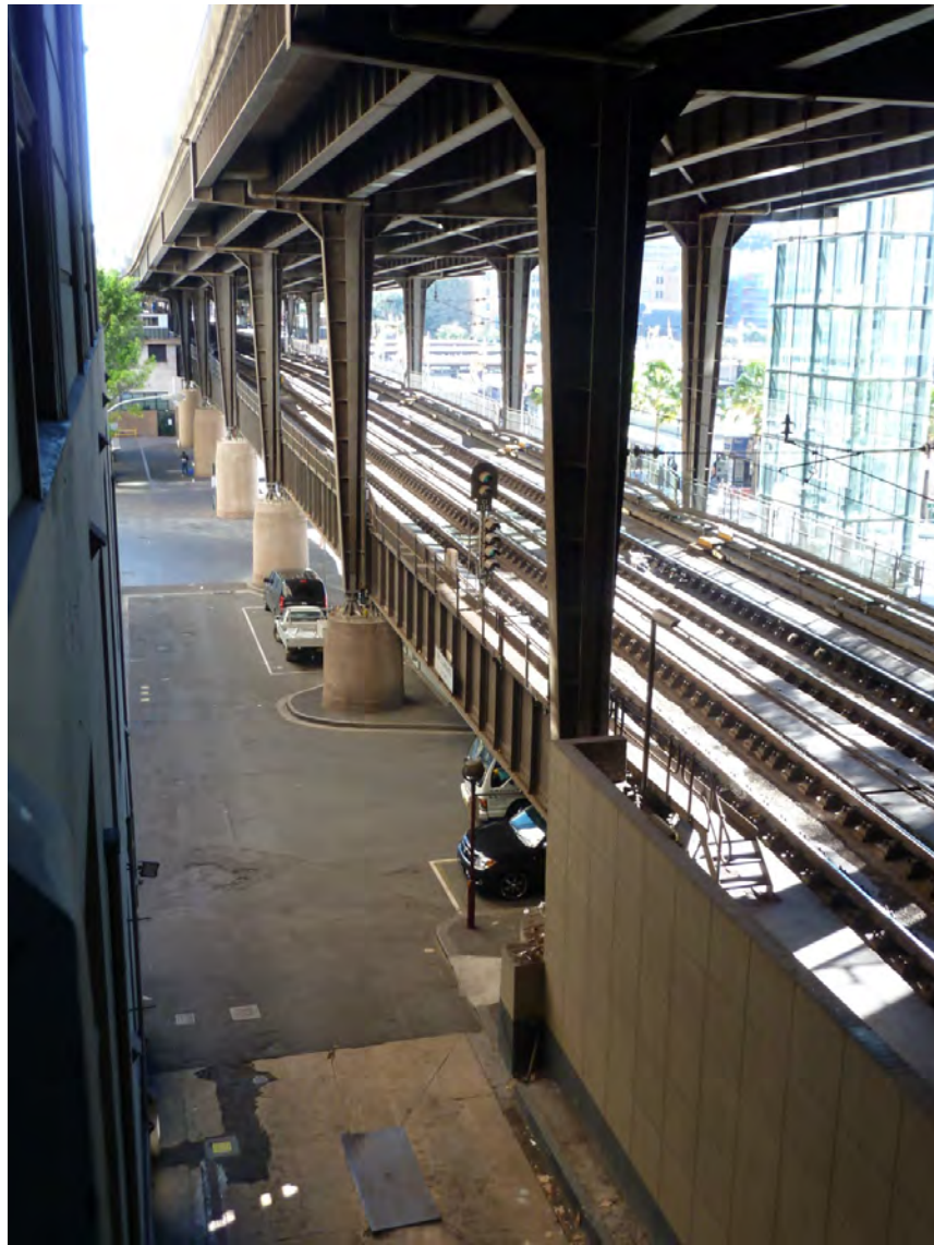
Figure 13 – Access road and rail viaduct, with the Cahill Expressway above
