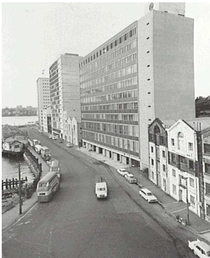
Figure 2.9: Photograph of part of the four sandstone warehouses located at 71-79 Macquarie Street showing their East Circular Quay frontage, taken in 1962 just prior to their demolition. (Source: City of Sydney Archives, Citation: 026\026626).
