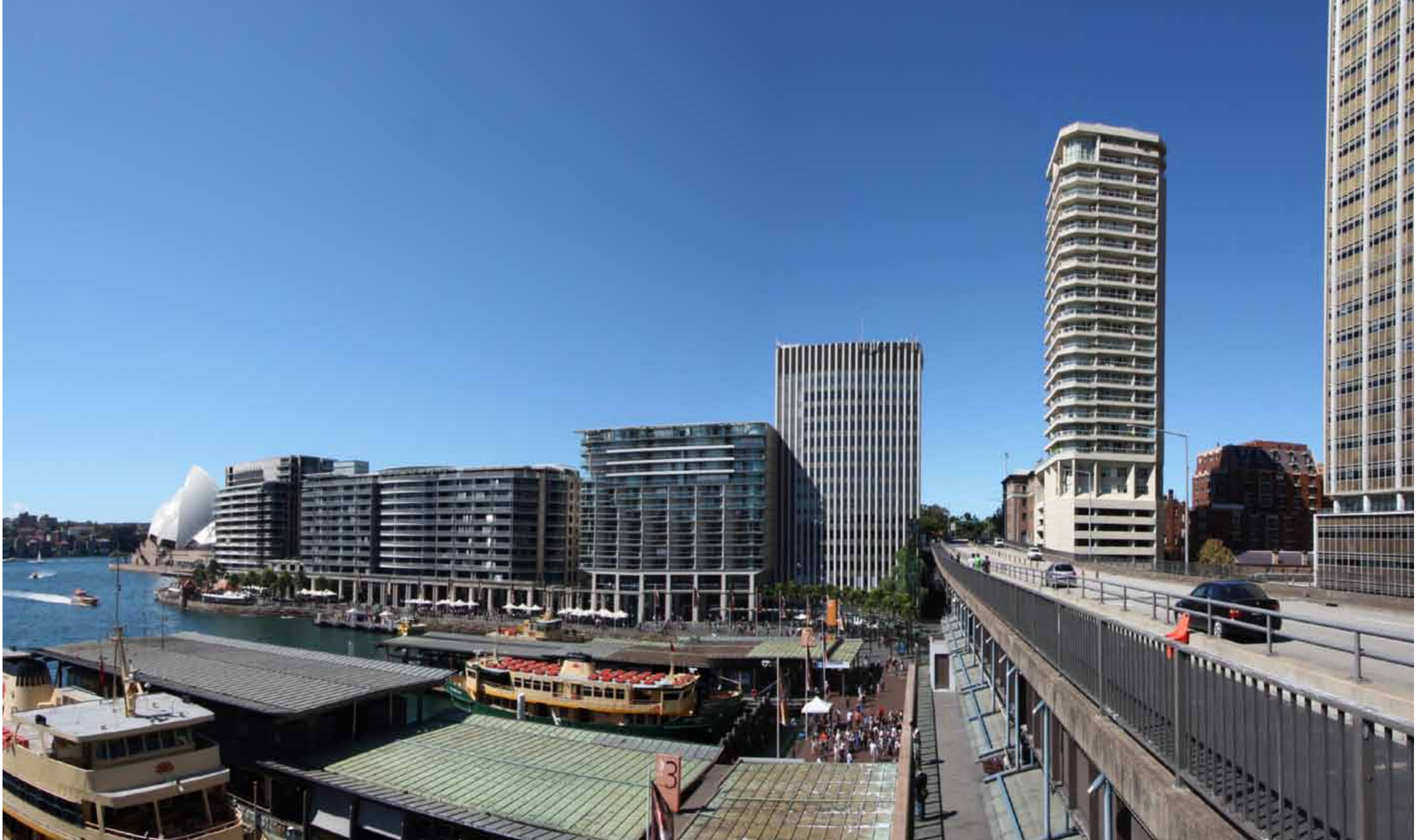
Existing Building, Western Facade Viewed from The Cahill Expressway
