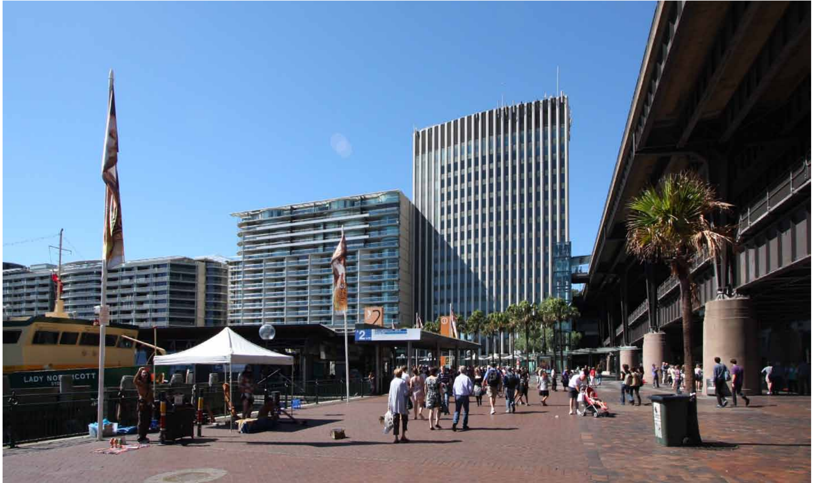
Existing Building, Western Facade Viewed from Circular Quay
