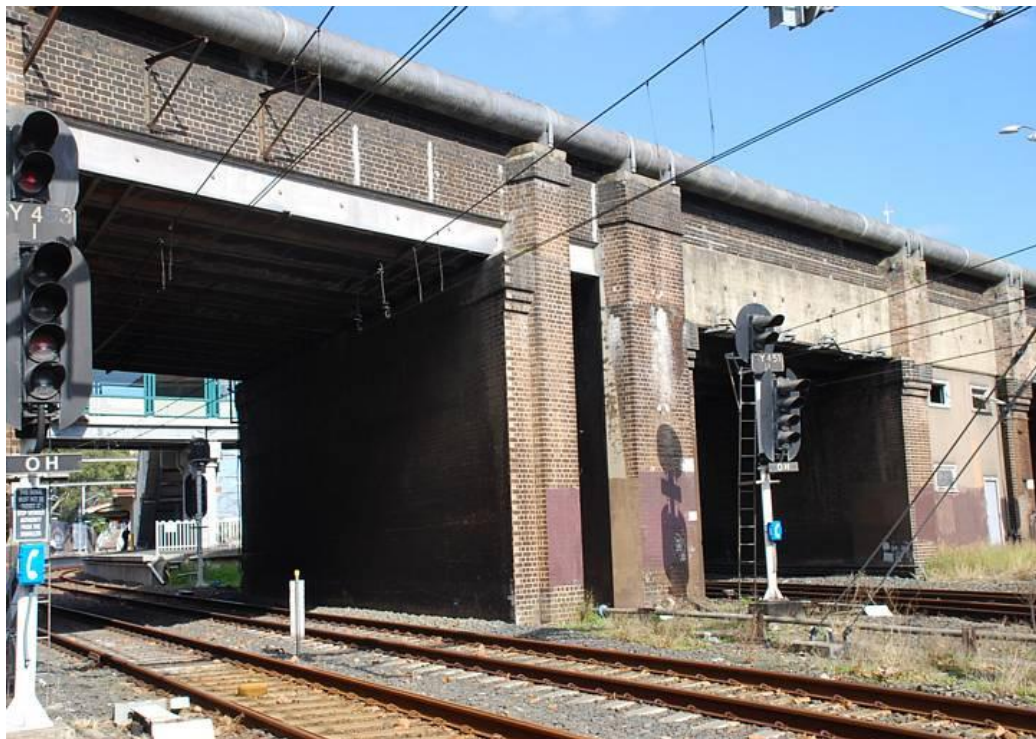
Figure 10 - North face of Lawson Street Overbridge, c200?
