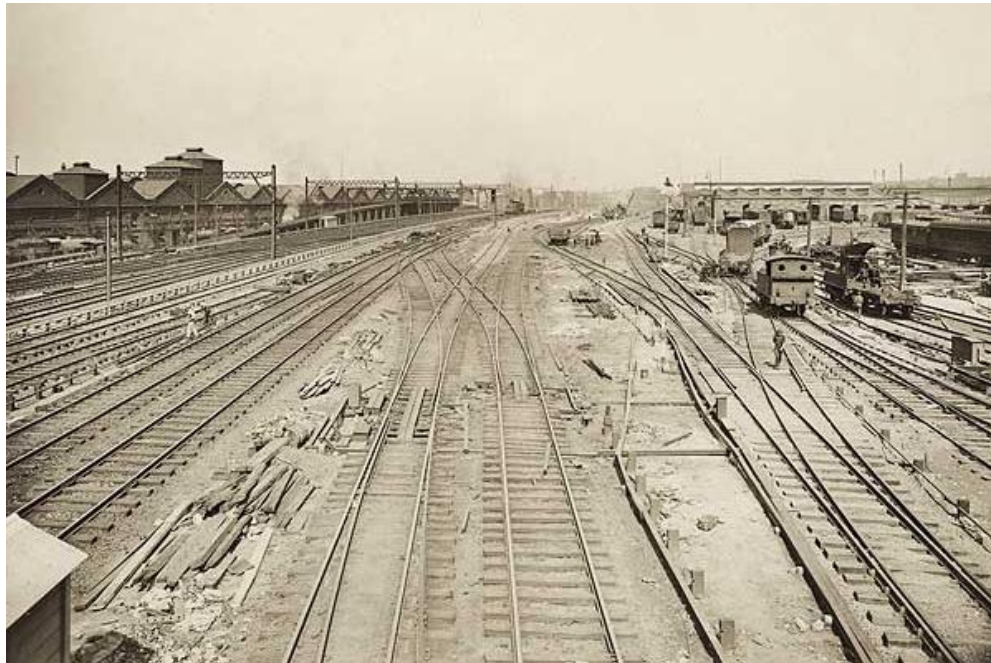
Figure 7 - Illawarra Steam Dive under construction - view from Workmen's Footbridge Eveleigh looking west, undated.
