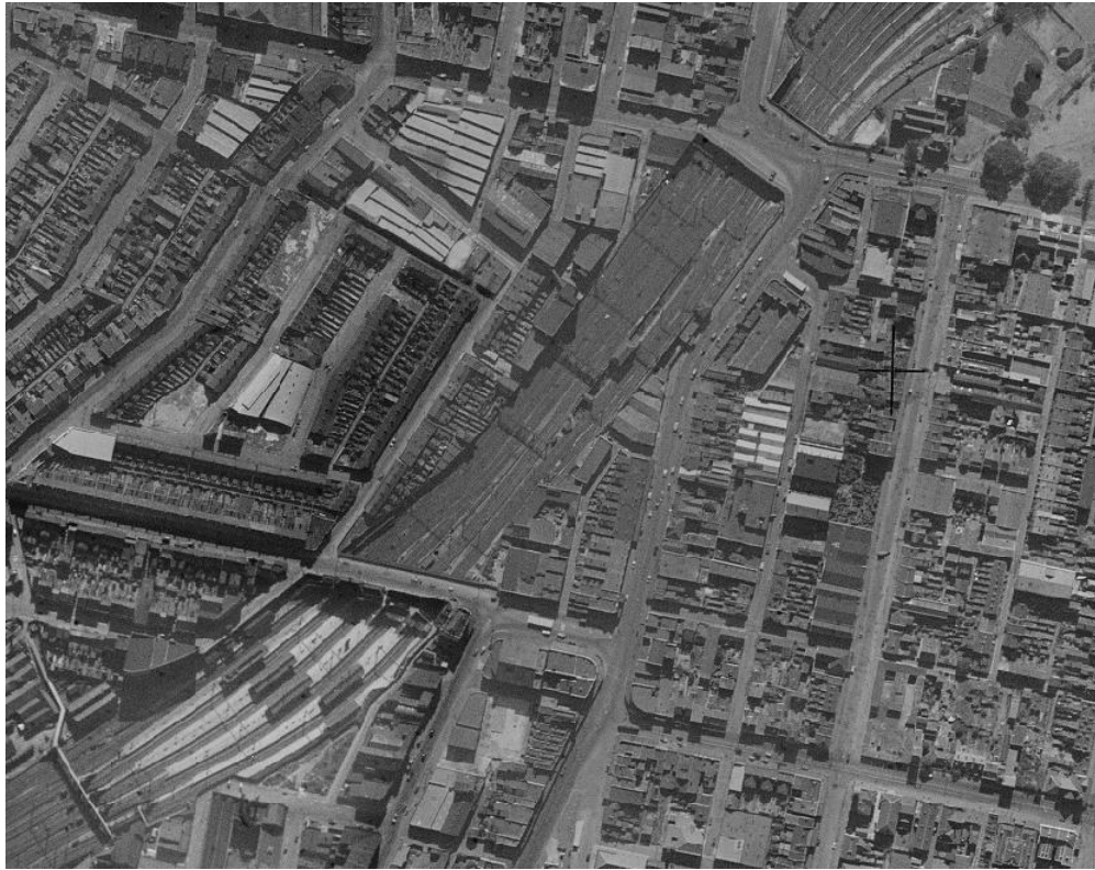
Figure 13 - 1943 aerial of Redfern, Eveleigh and Darlington illustrating the densely populated nature of the area and the location of various factory buildings.
