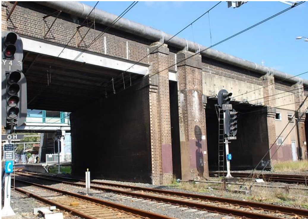
Figure 11 - North face of Lawson Street Overbridge, 2000s (Source: State Heritage)
