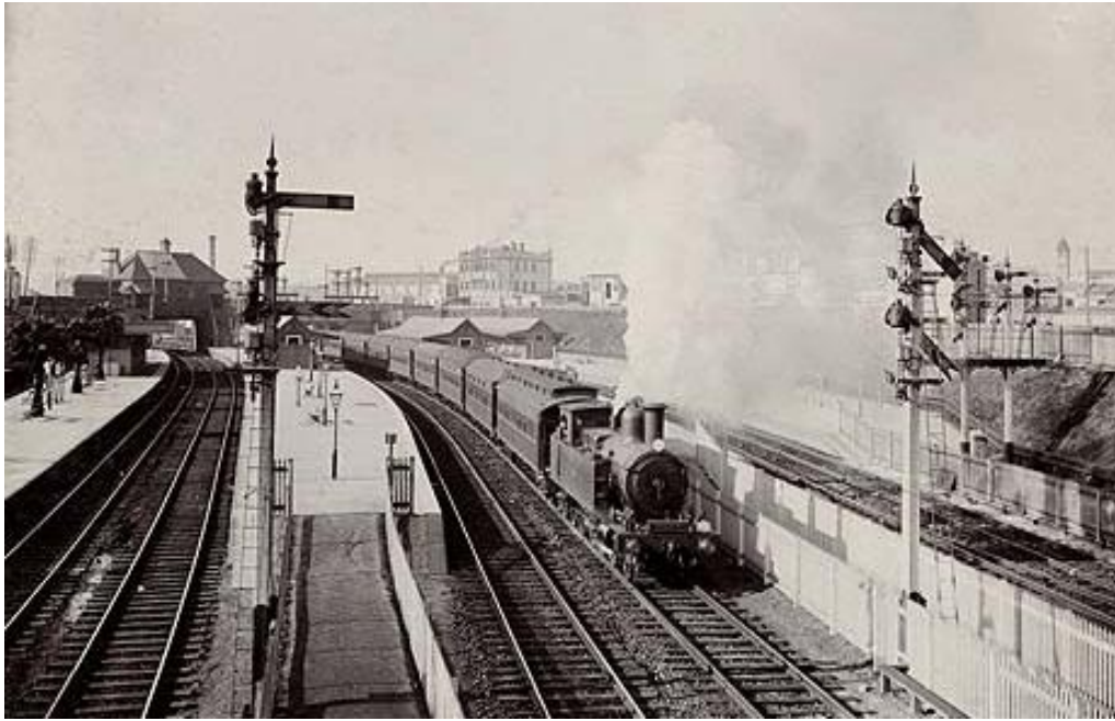
Figure 9 - View of Redfern Railway Station, undated. Source: 878/20, State Records
