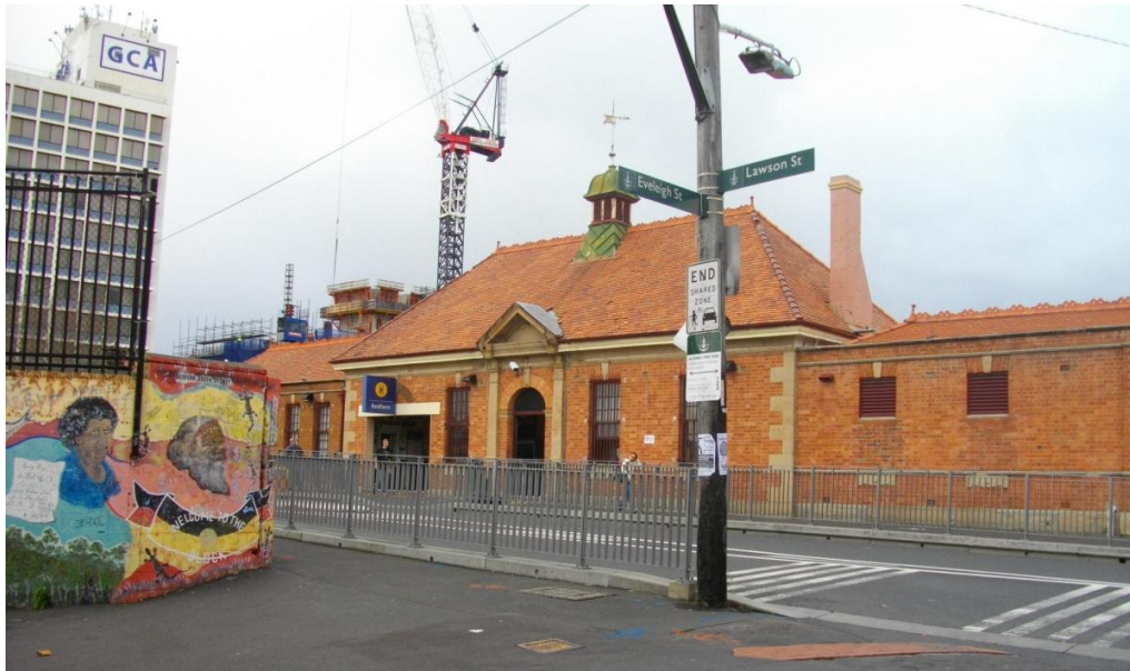
Figure 25 – View from the corner of Eveleigh and Lawson Streets looking southeast to the Queen Anne style, Redfern Station, listed as a State significant heritage item as part of the Redfern Railway Station Group that dates to 1891 (Source: NBRSPARTNERS, June 2011)
