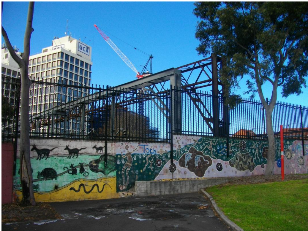
Figure 24 – View east from Eveleigh Street, showing the blockwork wall with metal palisade fence over, located above the retaining wall. The blockwork wall is painted with murals by the Aboriginal community and date to the 1990s. Overhead wire infrastructure is visible beyond the fence (Source: NBRSPARTNERS, July 2011)
