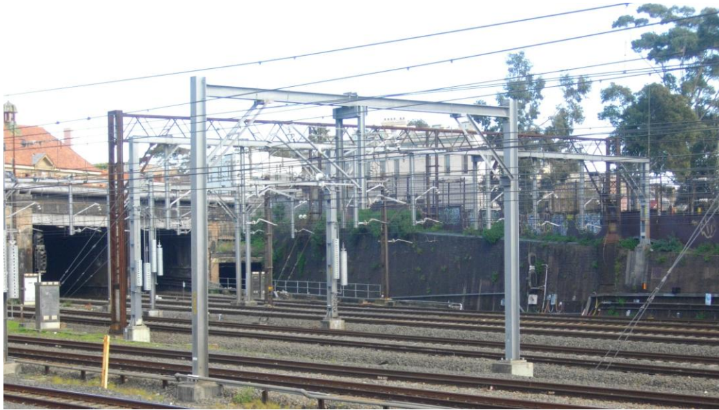
Figure 19 – View west from Gibbons Street across the tracks to the rail corridor retaining. The retaining wall gradates down from north to south, Services are mounted at the base of the retaining wall (Source: NBRS+PARTNERS, July 2011)
