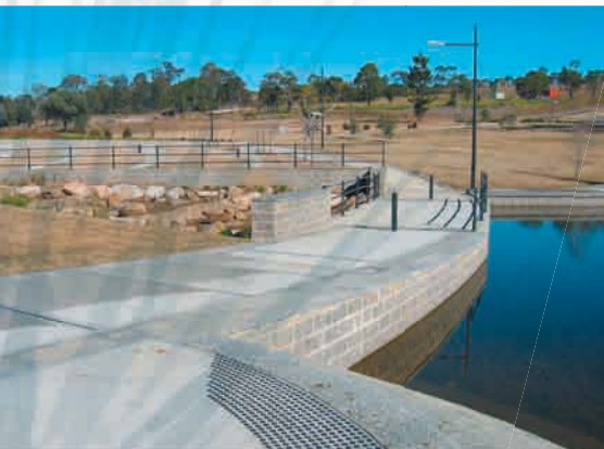
Hard edge treatment incorporating masonry walls and handrails.
