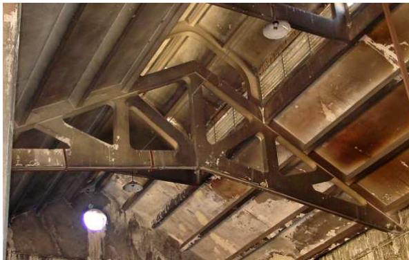
Reinforced concrete roof truss inside the Power House
