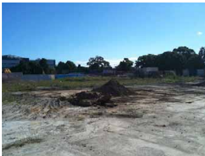
Figure 3. Layer of gravel covering concrete cap in Area 2.
