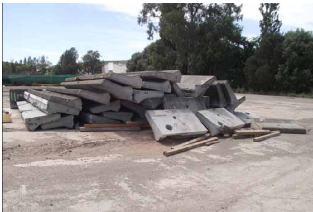
Plate 2: Concrete panels temporarily stockpiled in the west survey area.
