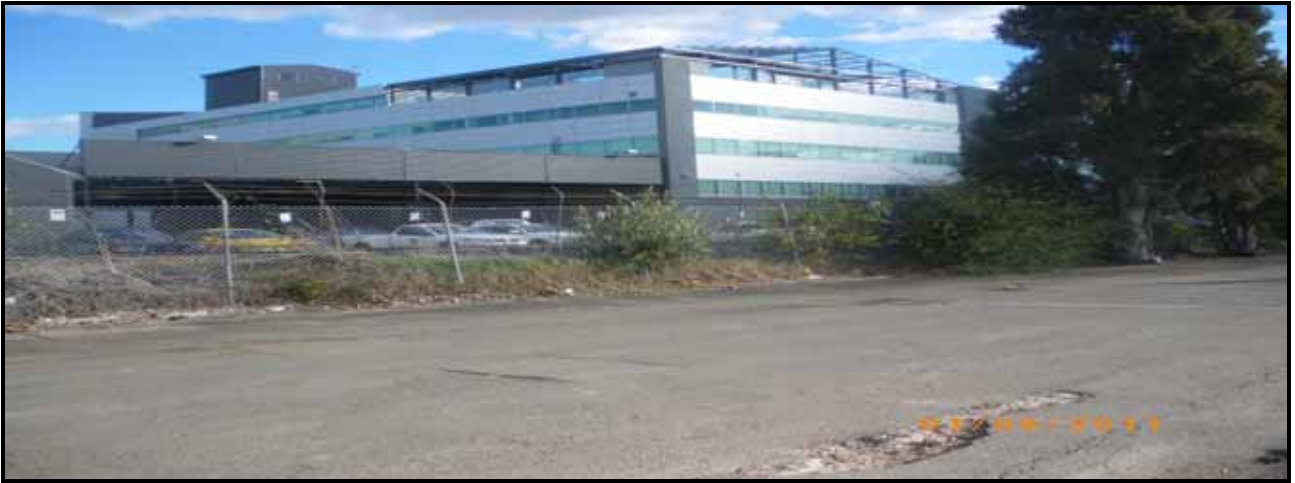
Plate 3.4 – View from the site of Aldi CarPark and Tilrox Building (including Child Care Centre) which are located to the south of the site.
