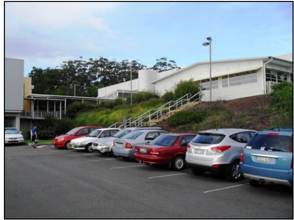
Photo 18 – Batter Slope to West of Car Park
