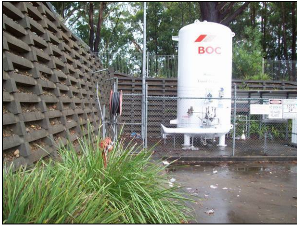
Photo 17 – Crib Wall in South West Site
