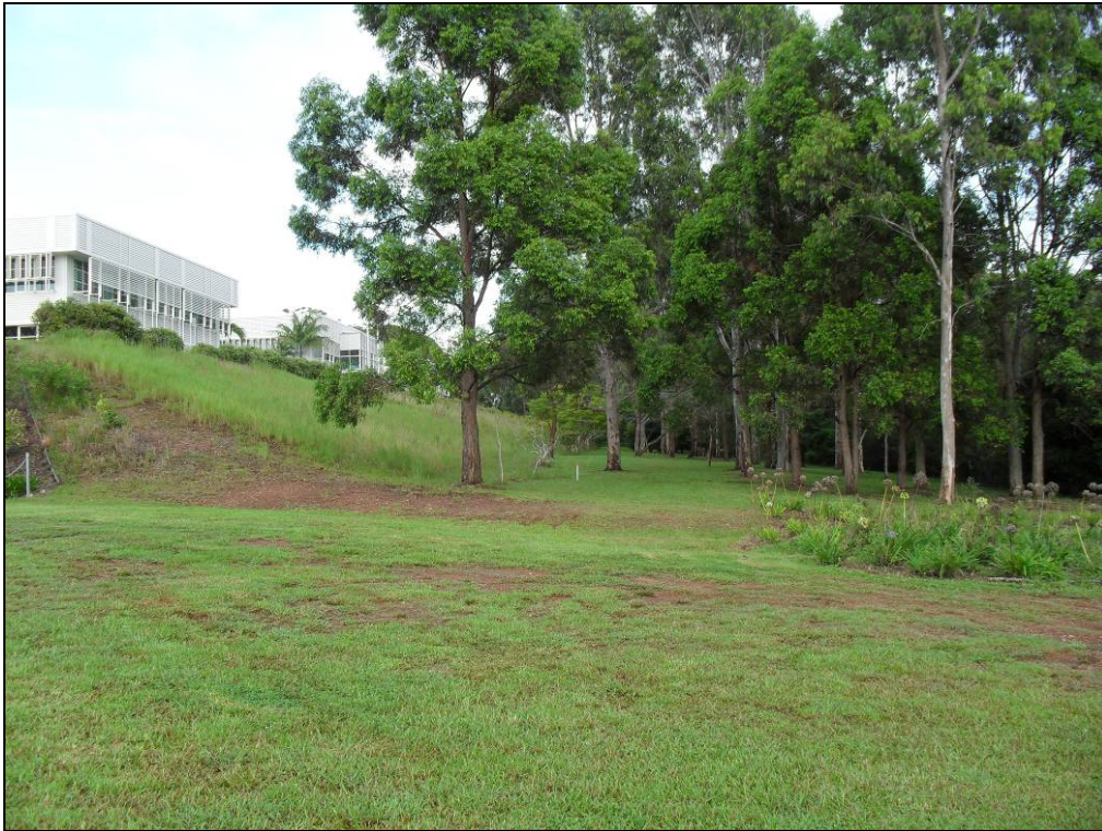
Photo 9: Looking west at fill embankment
