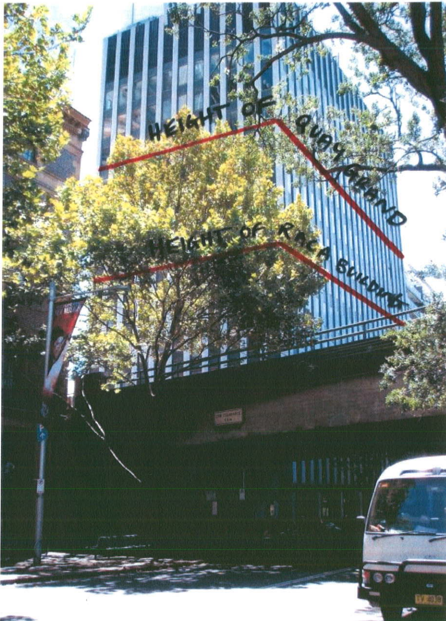
Figure 2 – Existing building’s inconsistency with street wall height.
