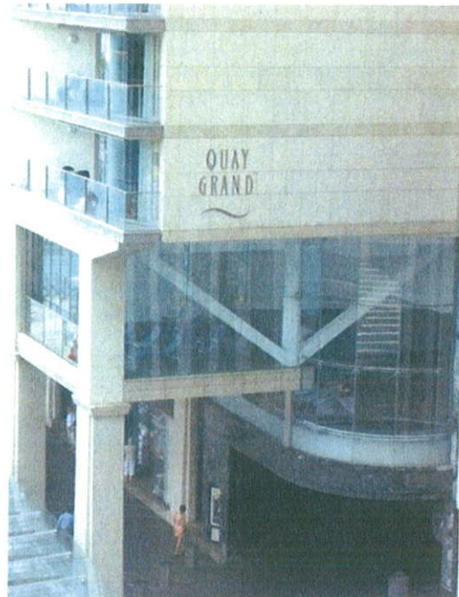
Photo 4: Pool area, view from Cahill Expressway Walkway
