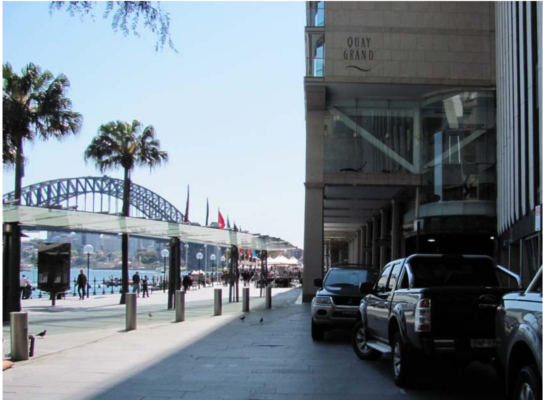
Figure 3: The Concept Plan will see the removal of all remaining vehicular traffic from East Circular Quay.
