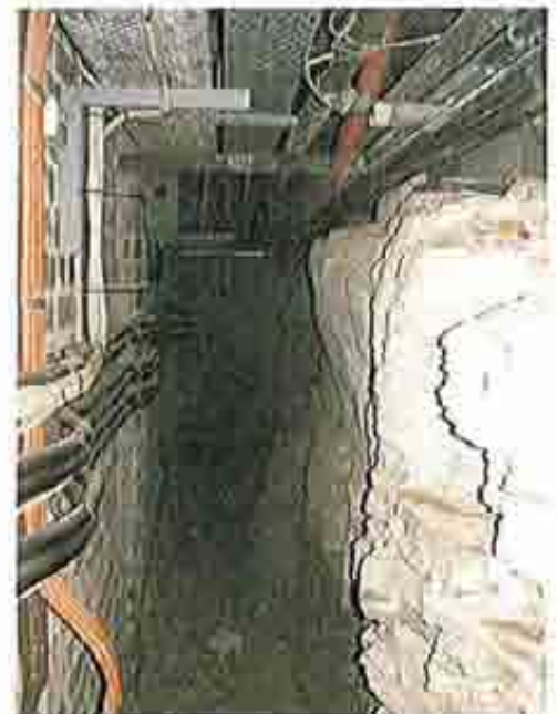
Photo 3: The footing access area for the basement of Building 4. Note the shale located immediately beneath the footings and other service pipes/cables
