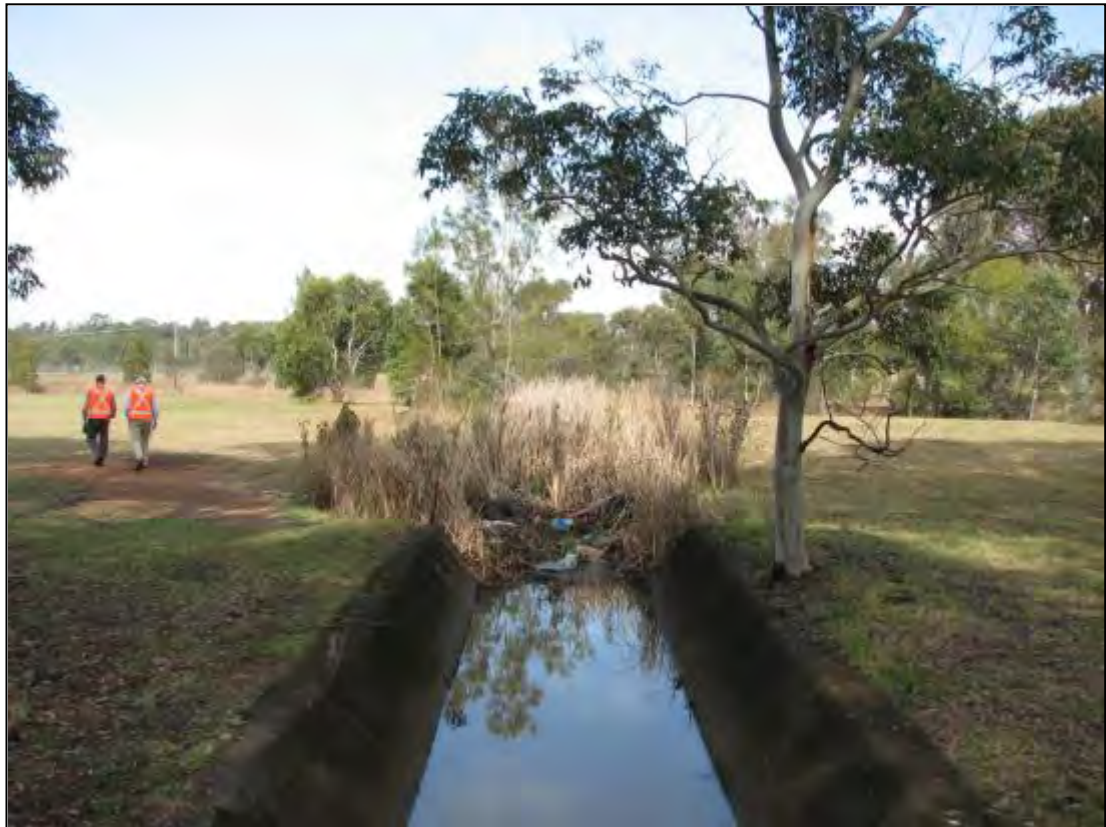
Photo shows concrete trapezoidal channel leading into heavily vegetated open channel which then drains to existing outlet on south-eastern corner
