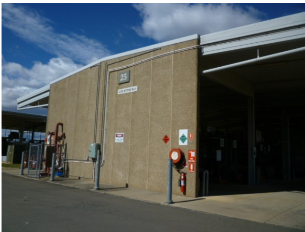
Figure 5: Example of building with reinforced concrete panels and steel roof
