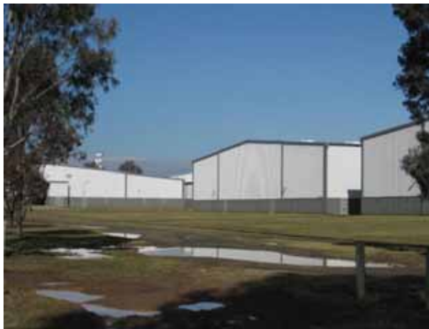
PICTURE 7 – EXISTING WAREHOUSE BUILDINGS
