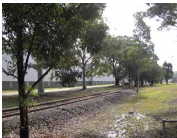
PICTURE 10 – EXISTING DISUSED RAIL LINE
