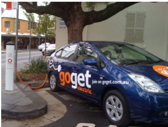
ABOVE Electric charging station at Glebe
