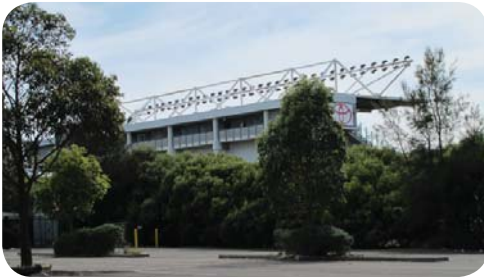
Carpark on western side of stadium
