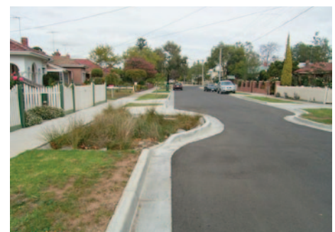
Bioretention to capture site stormwater runoff
