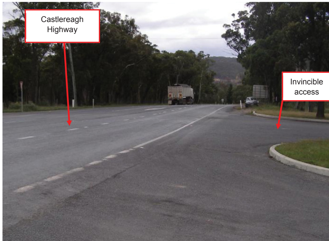
Figure 5-2 Entering sight distance from the Invincible access to the north.
