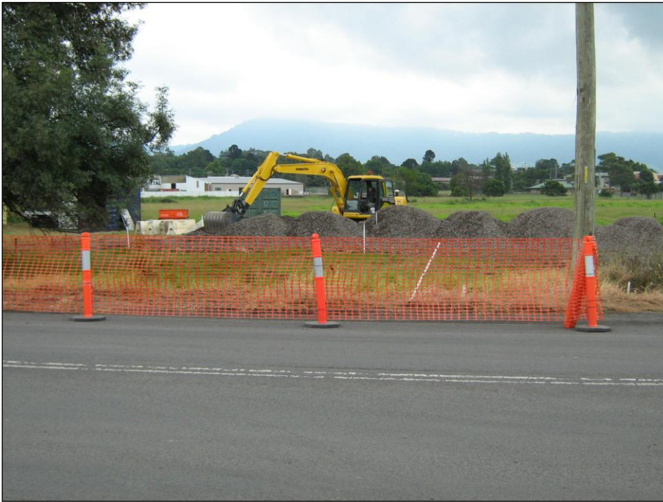
Plate 8. Construction in the Bolong Road survey area.
