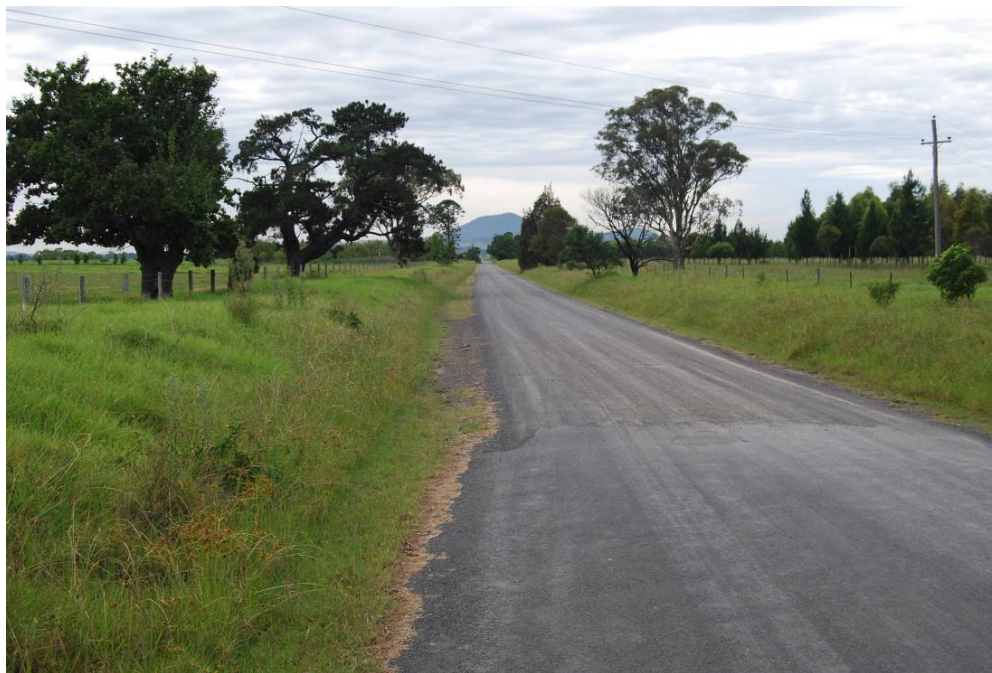
Photograph 3. Looking east along Fletchers Lane (route section D).
