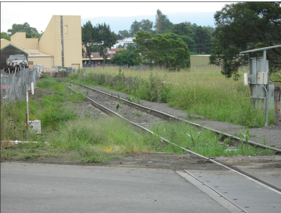
Plate 4. The existing rail line as it crosses Bolong Road.
