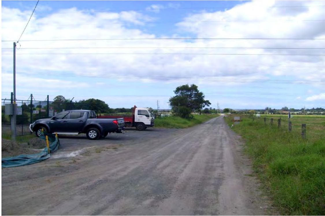
Photo 1 – Looking South-East Along Pestells Lane. The existing Eastern Gas Pipeline Transfer Station is shown to the left of frame
