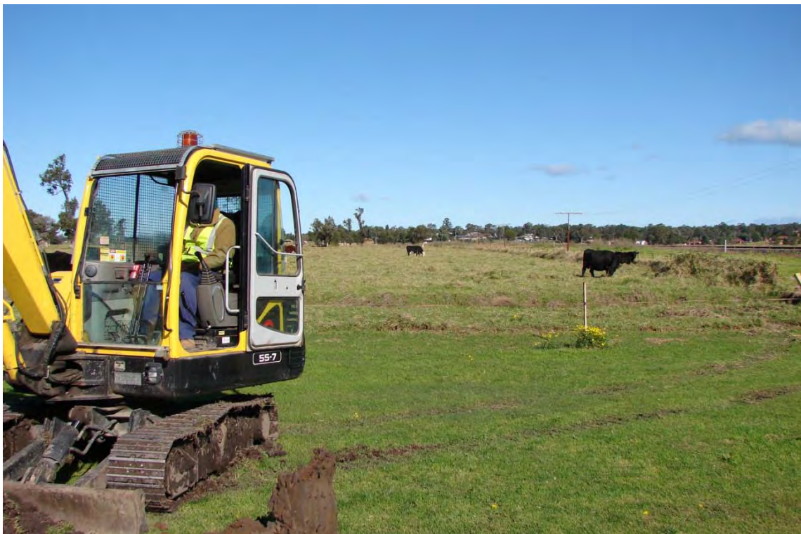
Photo 4 – Looking South Along SCC Owned Service Corridor and Manildra Owned Land
