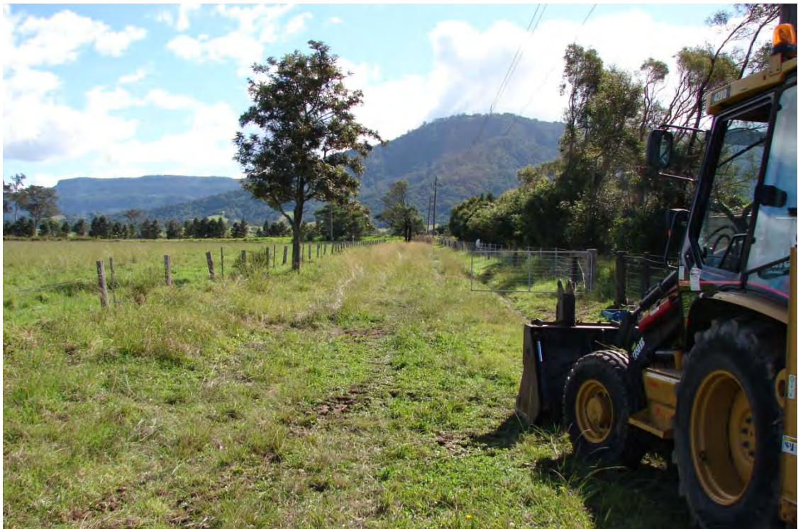
Photo 2 – Looking North-West Along Pestells Lane (SCC Owned Services Corridor)
