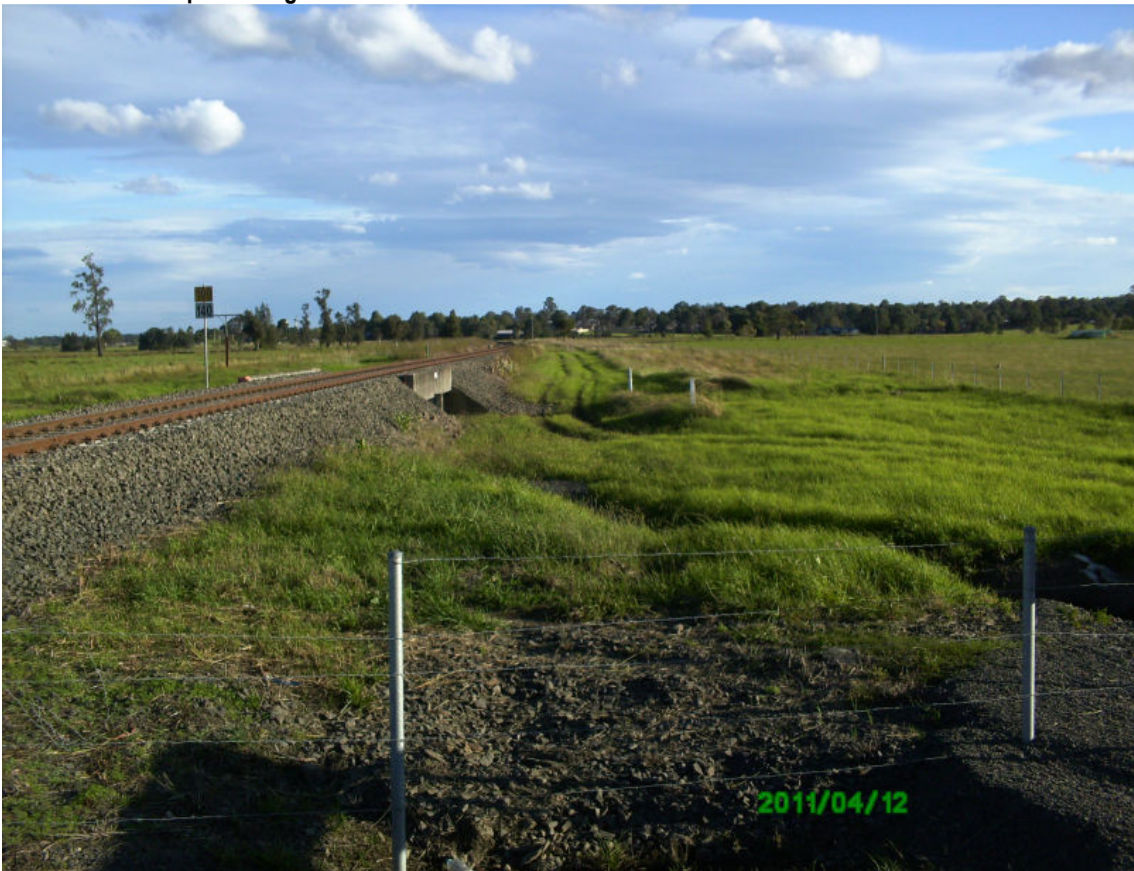
Photo 22-Large culvert in Railcorp railway reserve, beyond proposed railway track under-bore location
