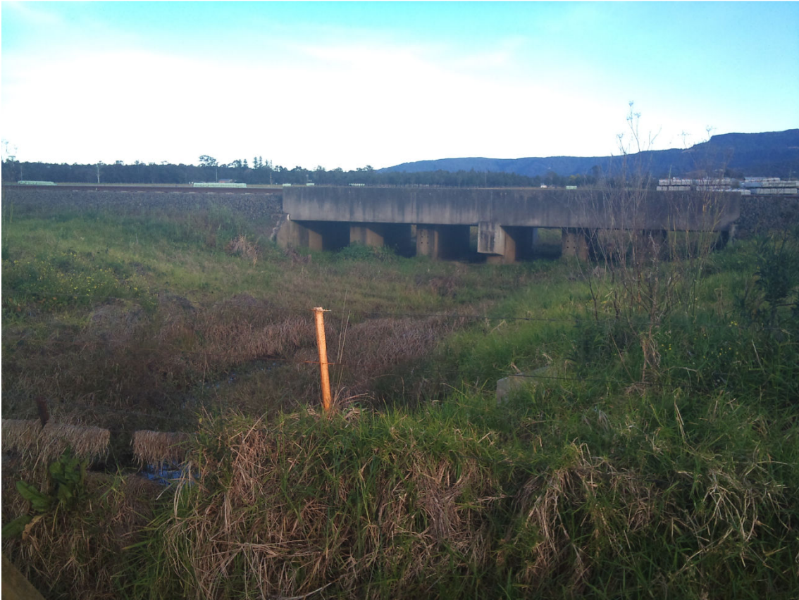
Photo 24b- First waterway crossing, showing culvert under railway tracks
