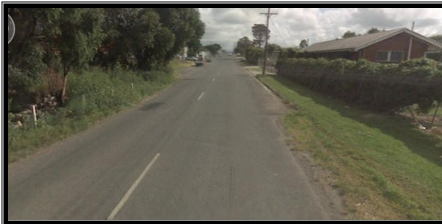
Railway Street looking north adjacent to the narrower section of carriageway restricted by the narrow western verge adjacent to the railway corridor.
