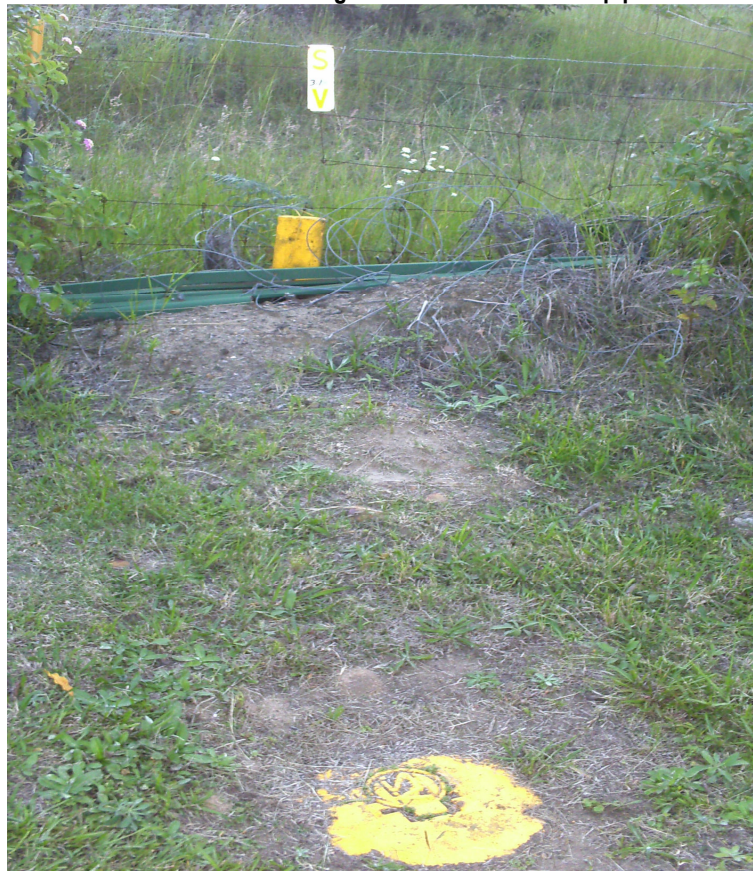
Photo 42- Water main infrastructure in Railway Street road reserve
