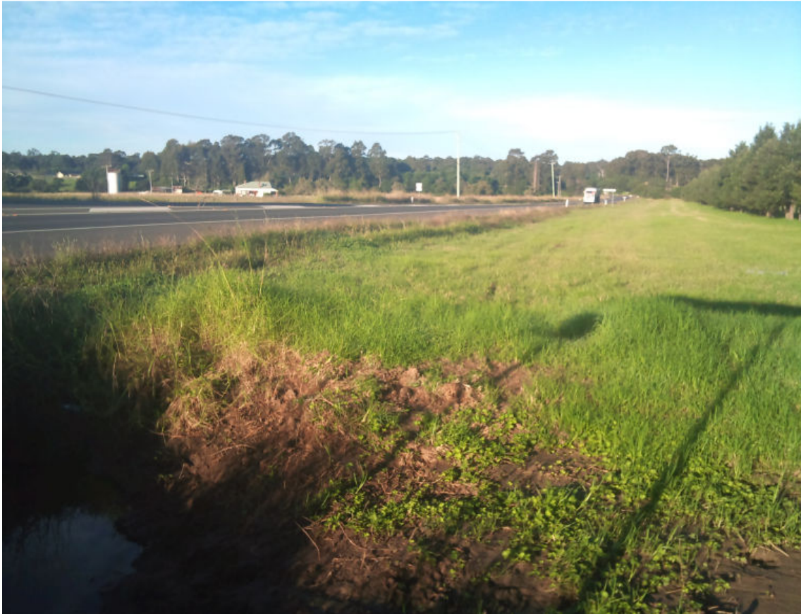
Photo 7- Table drain and culvert on Princes Highway intersection with Pestells Lane
