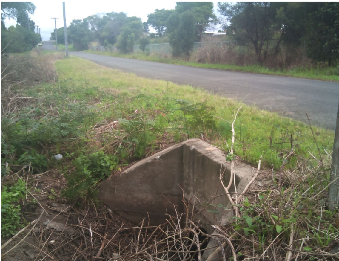
Photo 45- Stormwater headwall and culvert in Railway Street
