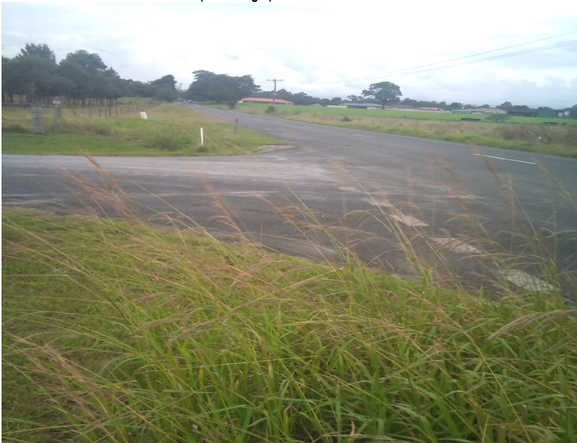
Photo 14-Fletchers Lane intersection with Meroo Road
