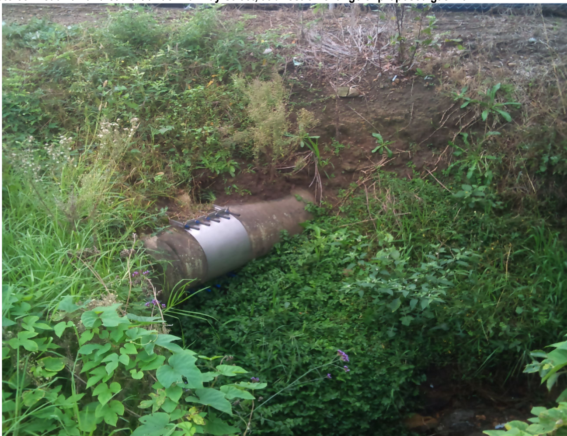
Photo 56- Sewer pipe through open channel drain in lot 1 DP825808
