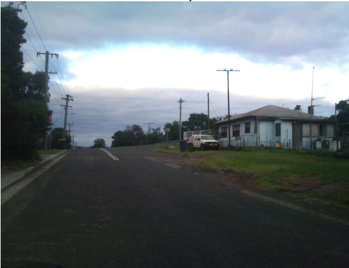
Photo 50- Looking at Cambewarra Road intersection with Railway Street
