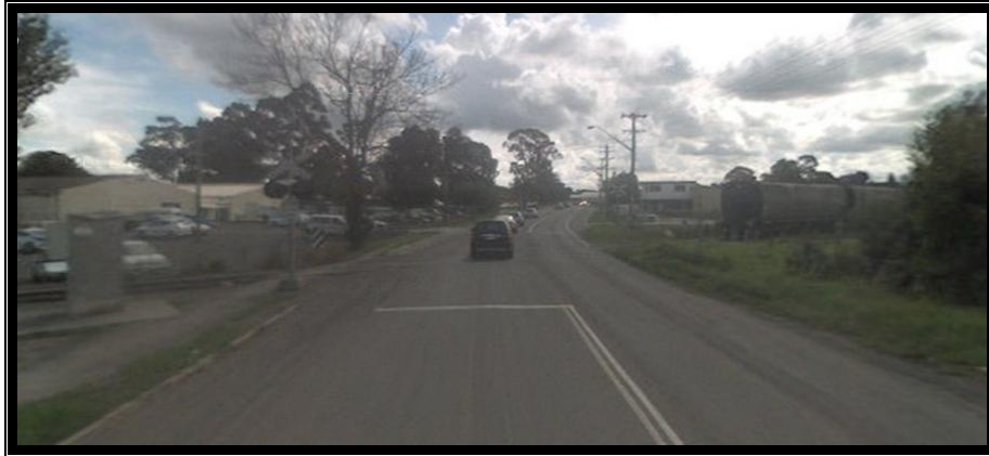
Bolong Road looking west to the Railway Corridor
