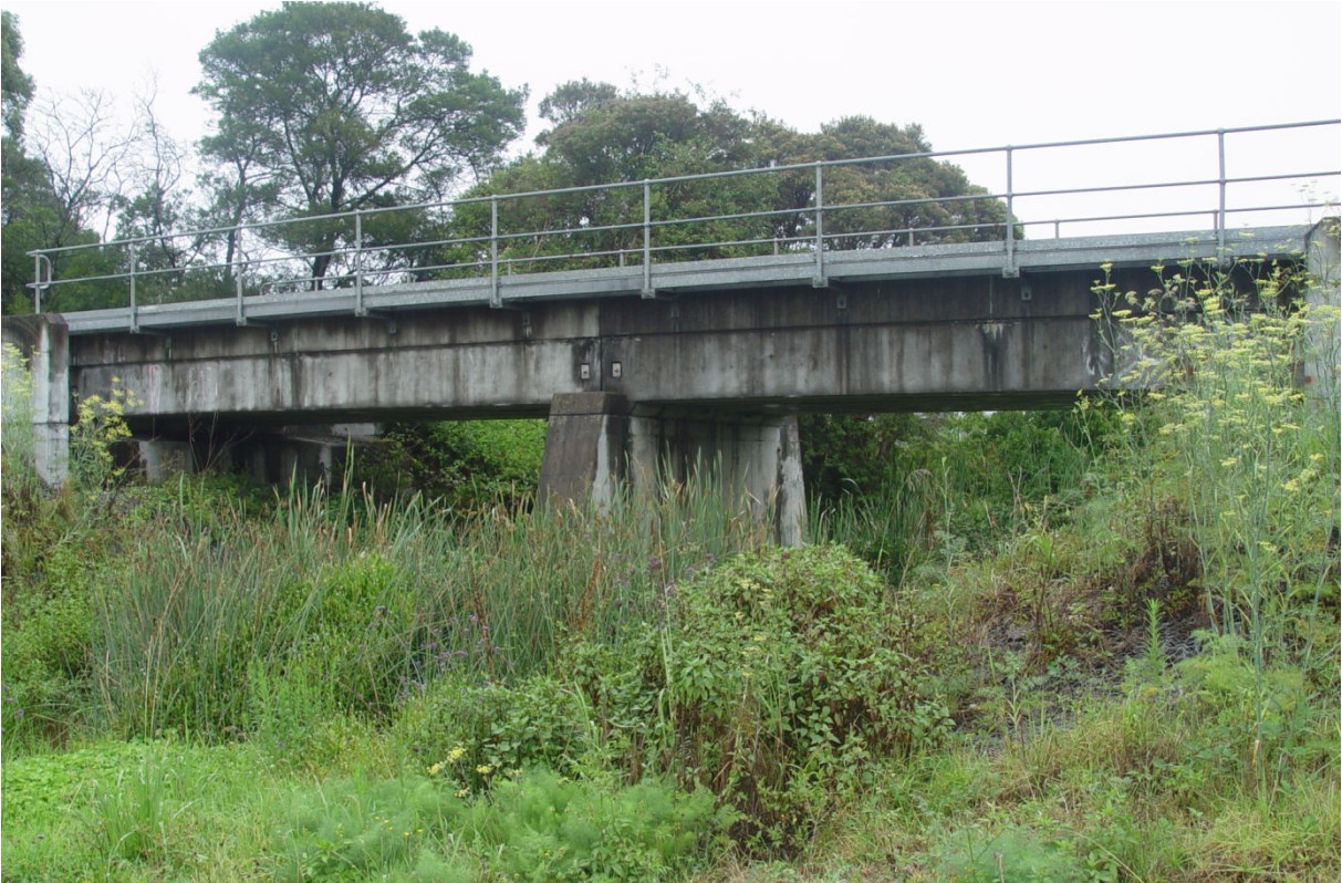
Figure 31: Large bridge #4 just upstream of waterway crossing 4.
