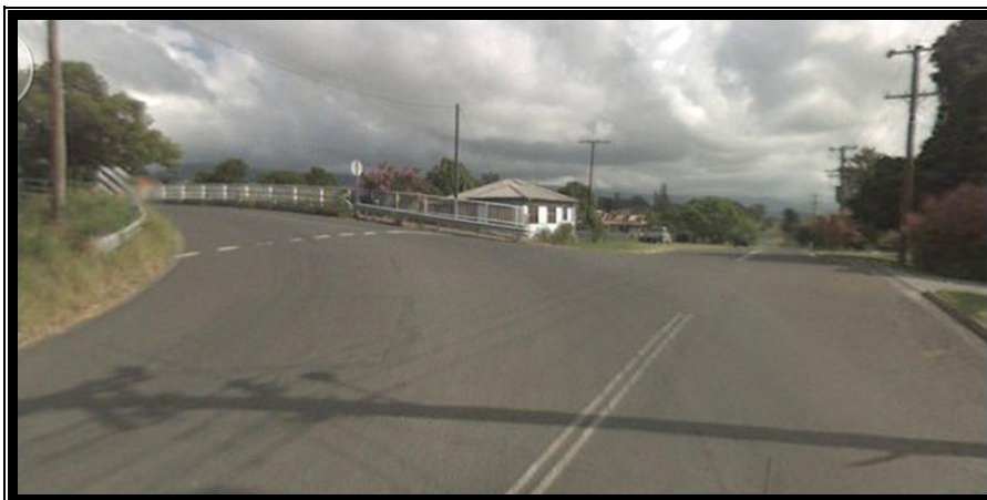
Railway Street & Cambewarra Road intersection – swept path for trucks from Cambewarra Road to Railway Street south would generally exclude the use of the kerbside (eastern) lane for the work-zone
