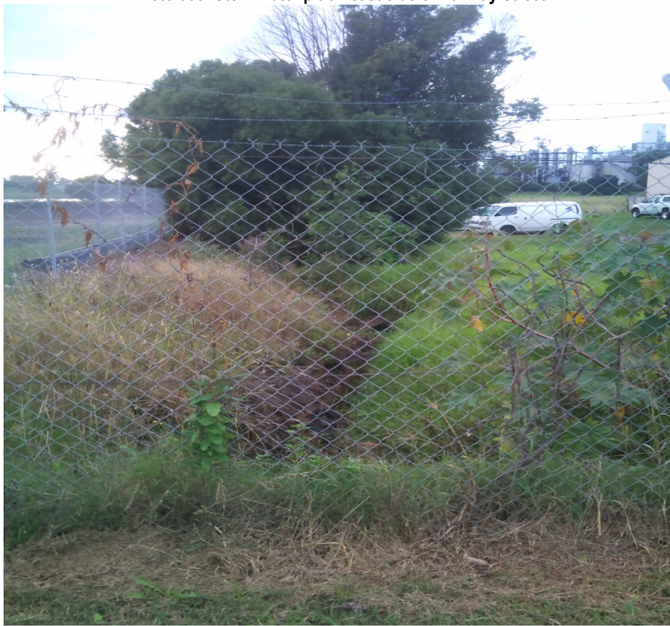
Photo 54- Open channel drain through lot 1 DP825808 Railway Street, taking water from pit shown in previous Photo.
