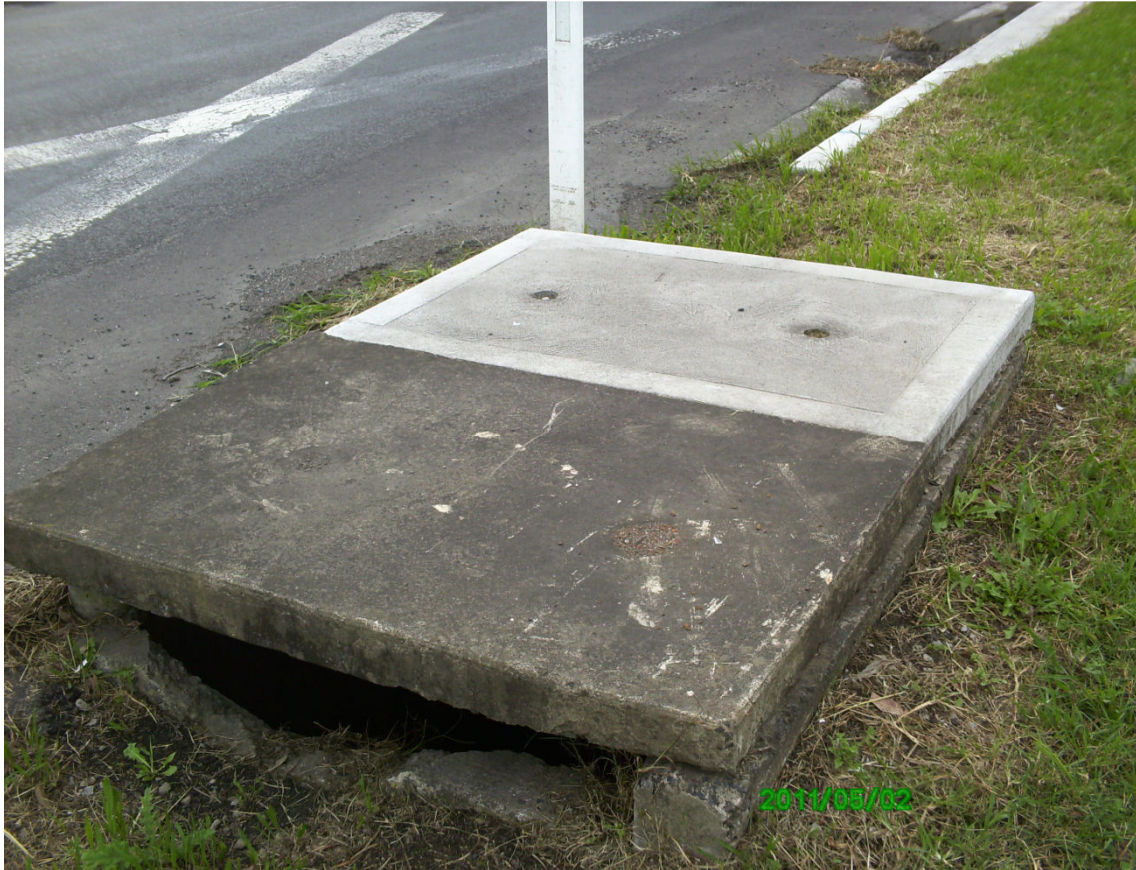
Photo 53c- Stormwater pit on east side of Railway Street
