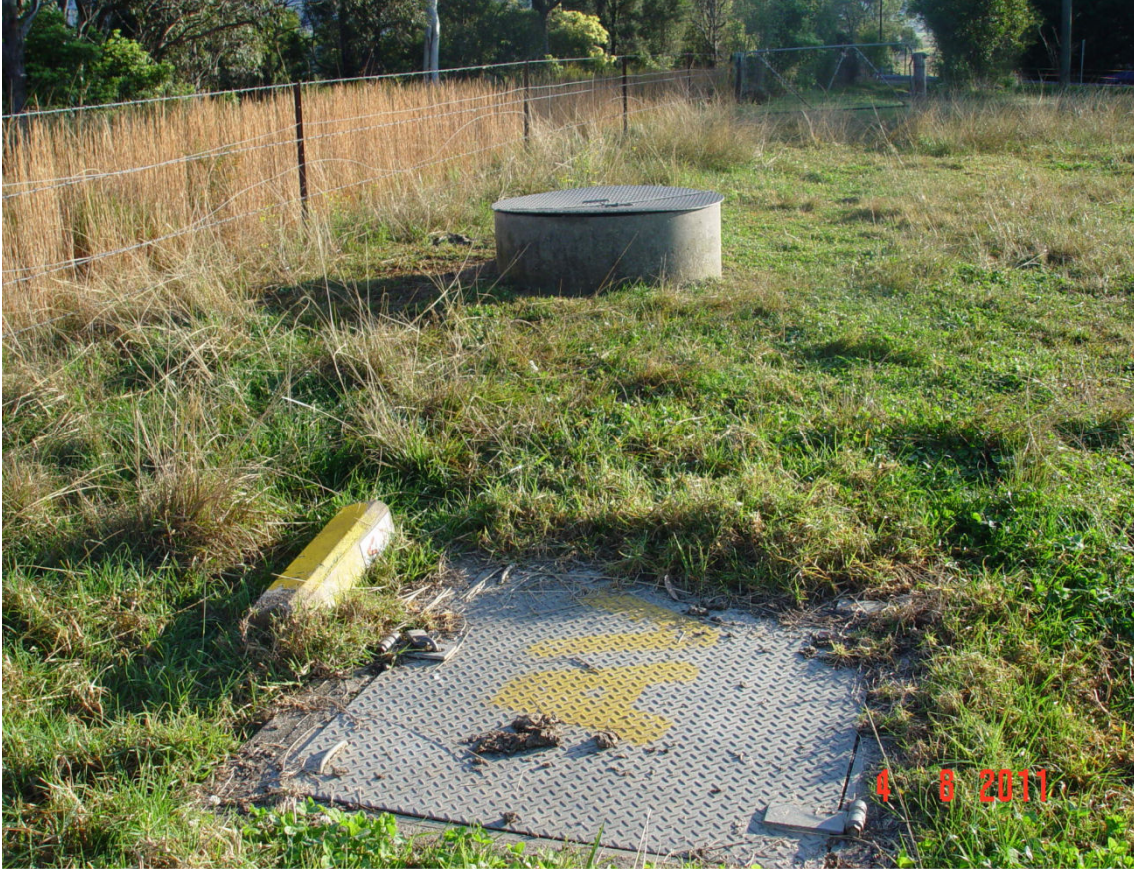
Photo 33- Water main infrastructure in un-named road reserve
