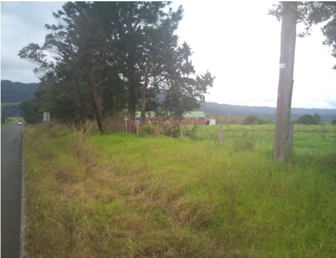
Photo 12-Table drain along Meroo Road
