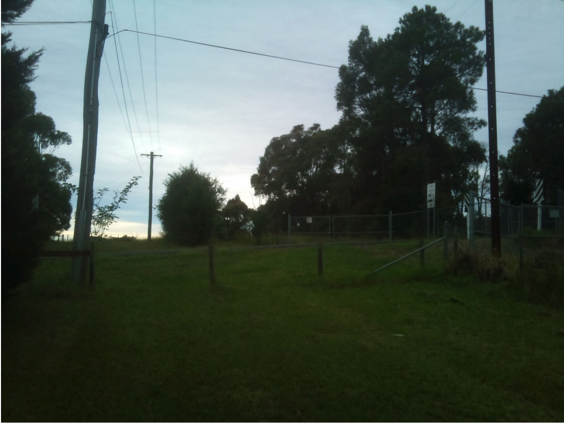
Photo 31- Edwards Avenue crossing point on north side
