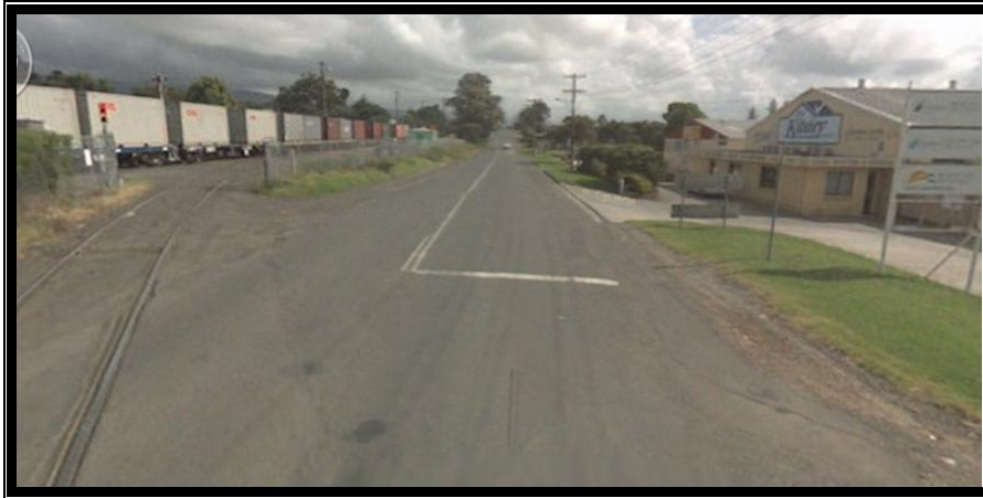
Railway Street looking north from outside the SSPL Packaging Place; note wide verge available
