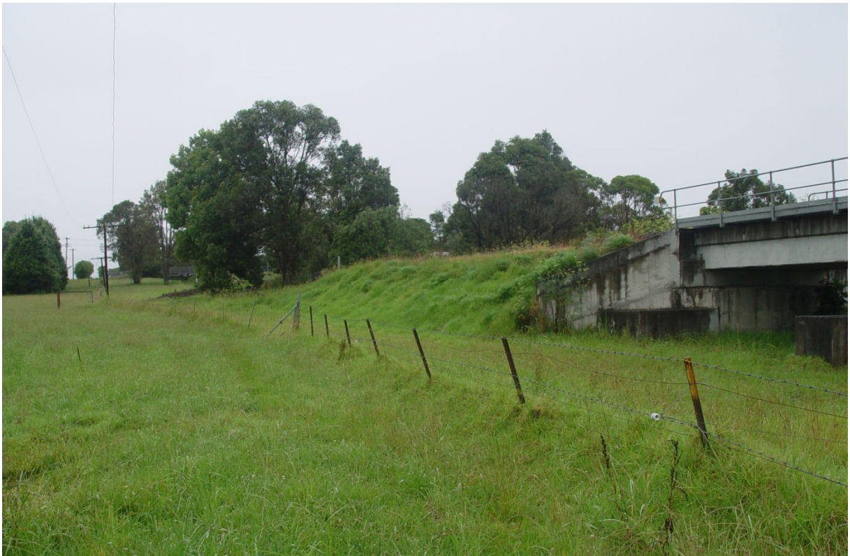
Figure 27: Looking south toward Edwards Avenue, at waterway crossing 3
