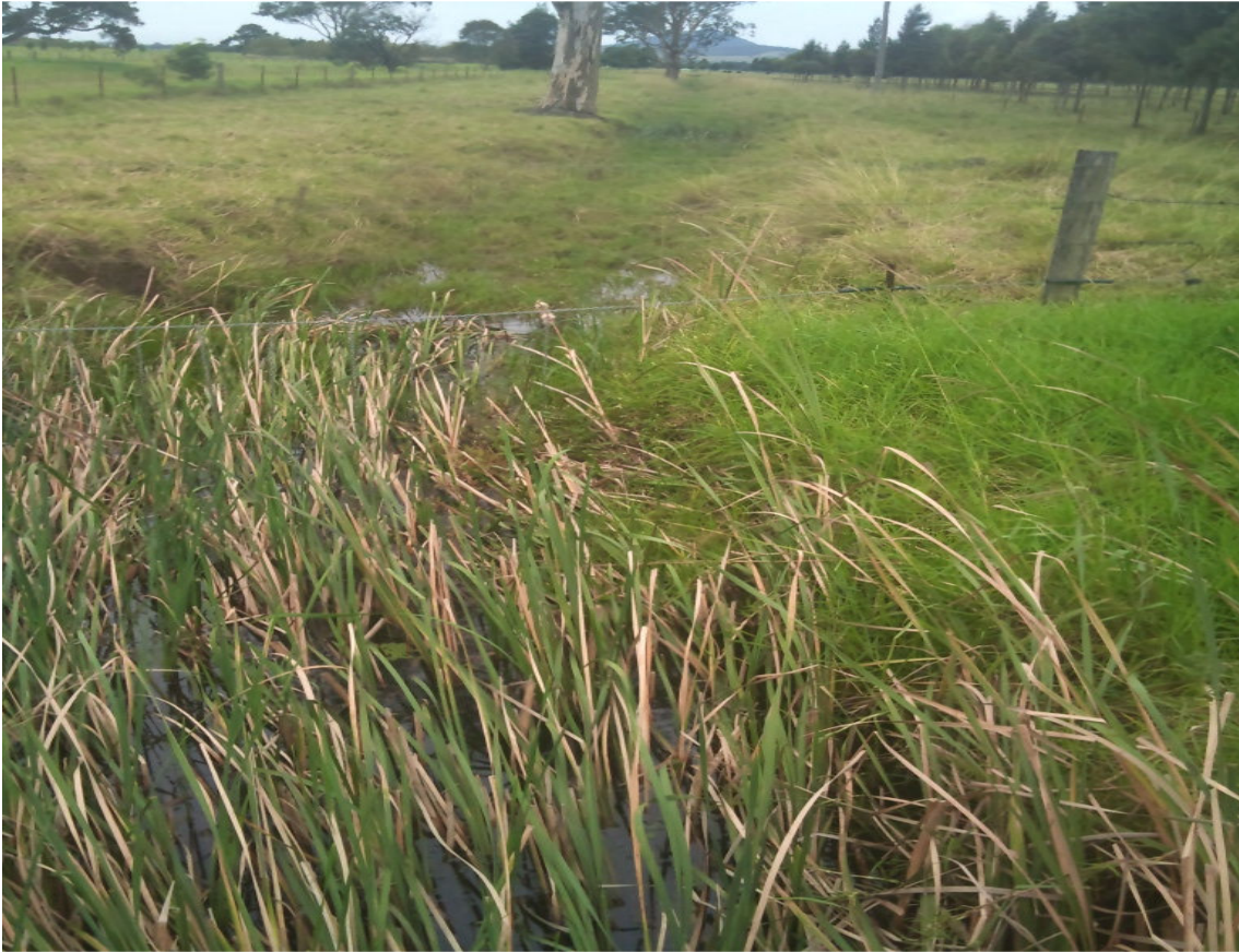
Photo 17-Open channel drain through paddock on south side of Fletchers Lane
