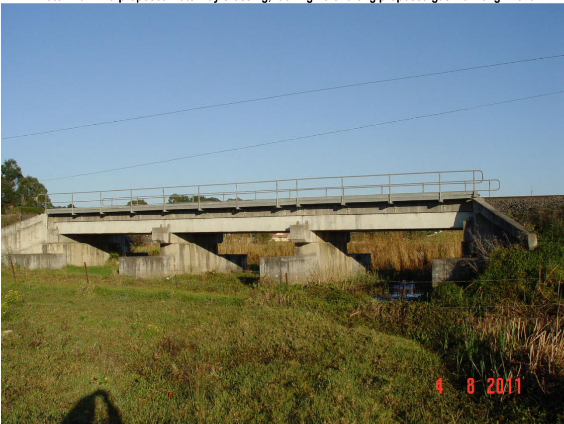
Photo 27c- Large railway bridge/culvert at third proposed waterway crossing
