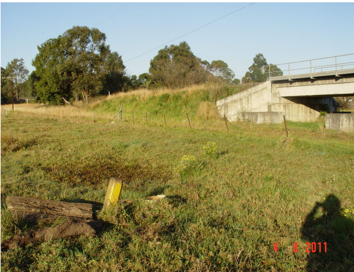
Photo 27a-Scour valve in un-named road reserve adjacent to third proposed waterway crossing, north of Edwards Avenue
