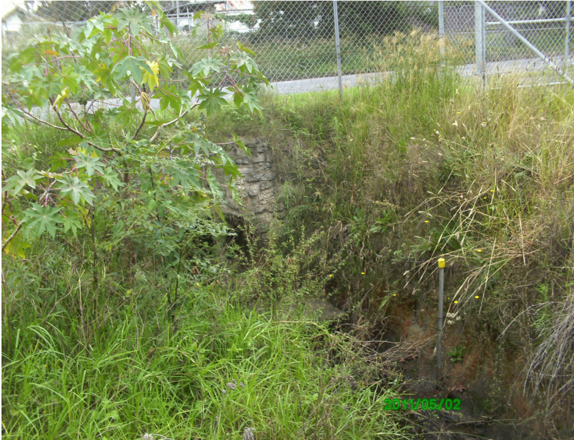
Photo 55- Headwall and culvert under Railway Street, at direction change of proposed gas main
