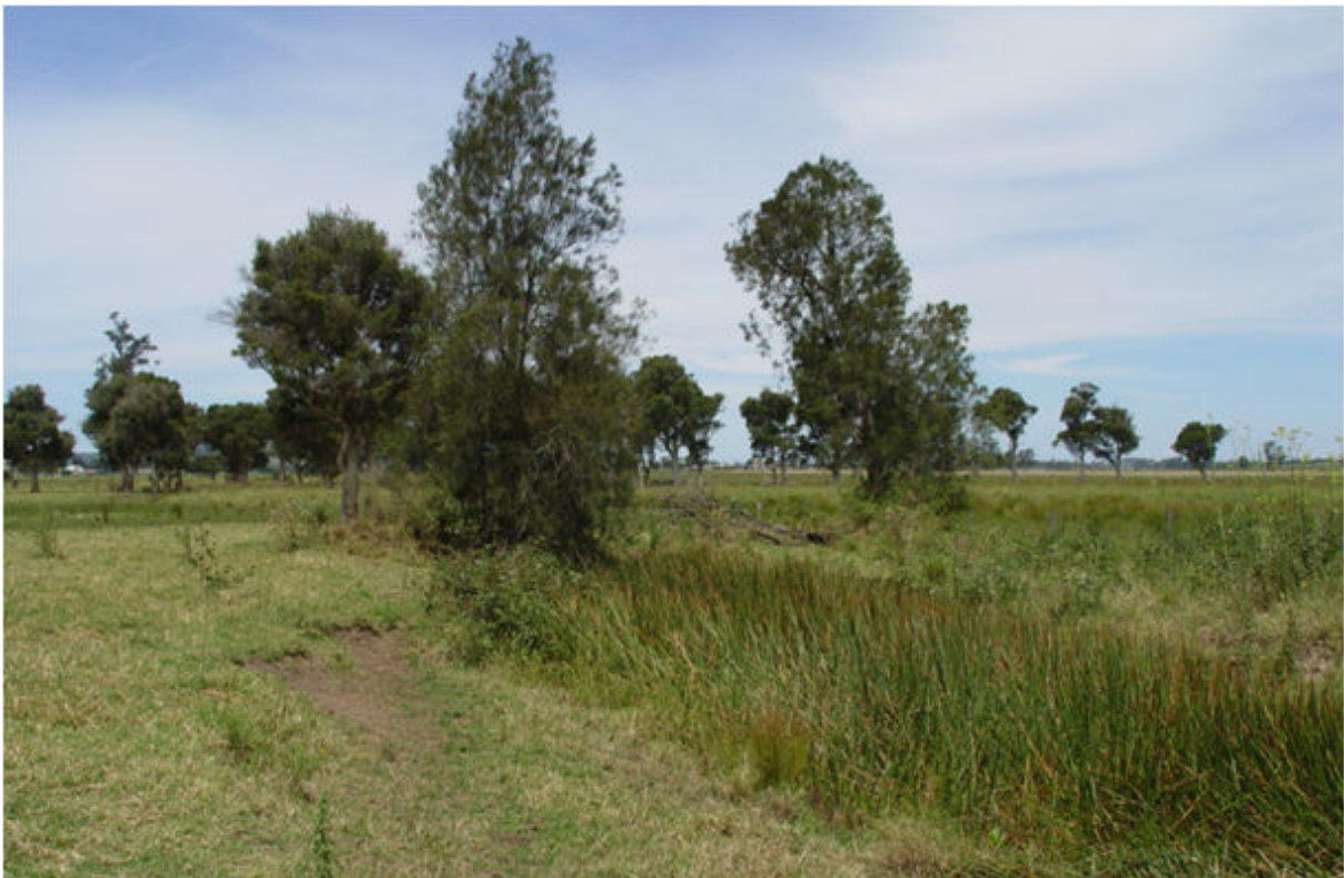
Figure 14: Bank Instability and Erosion at waterway crossing 2.
