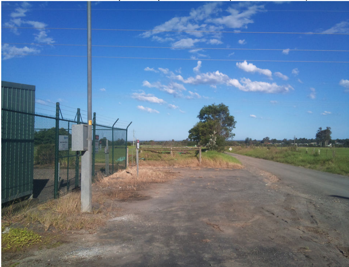
Photo 2 Eastern Gas Pipeline tie-in point for existing ActewAGL gas pipeline at Pestells Lane
