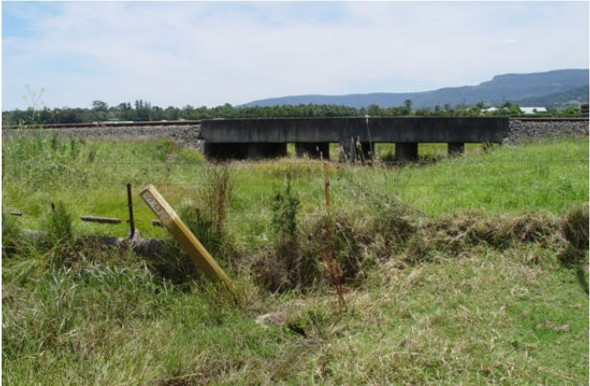
Figure 2: Culvert /Bridge #1 upstream of waterway crossing, and South of Fletchers Lane.
