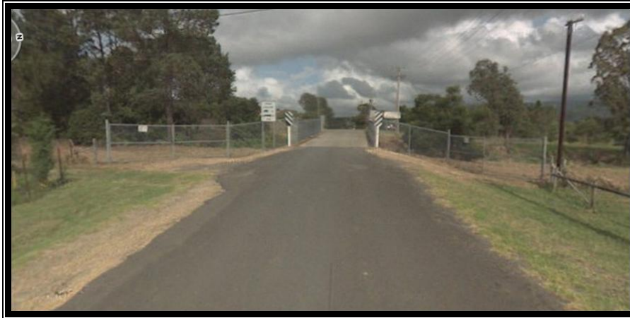
Edwards Avenue looking west towards narrow bridge over railway
