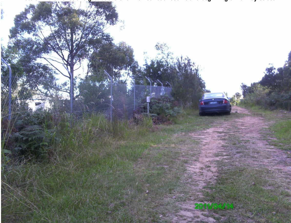
Photo 38- un-formed section of Railway Street, looking at ActewAGL existing gas main testing station
