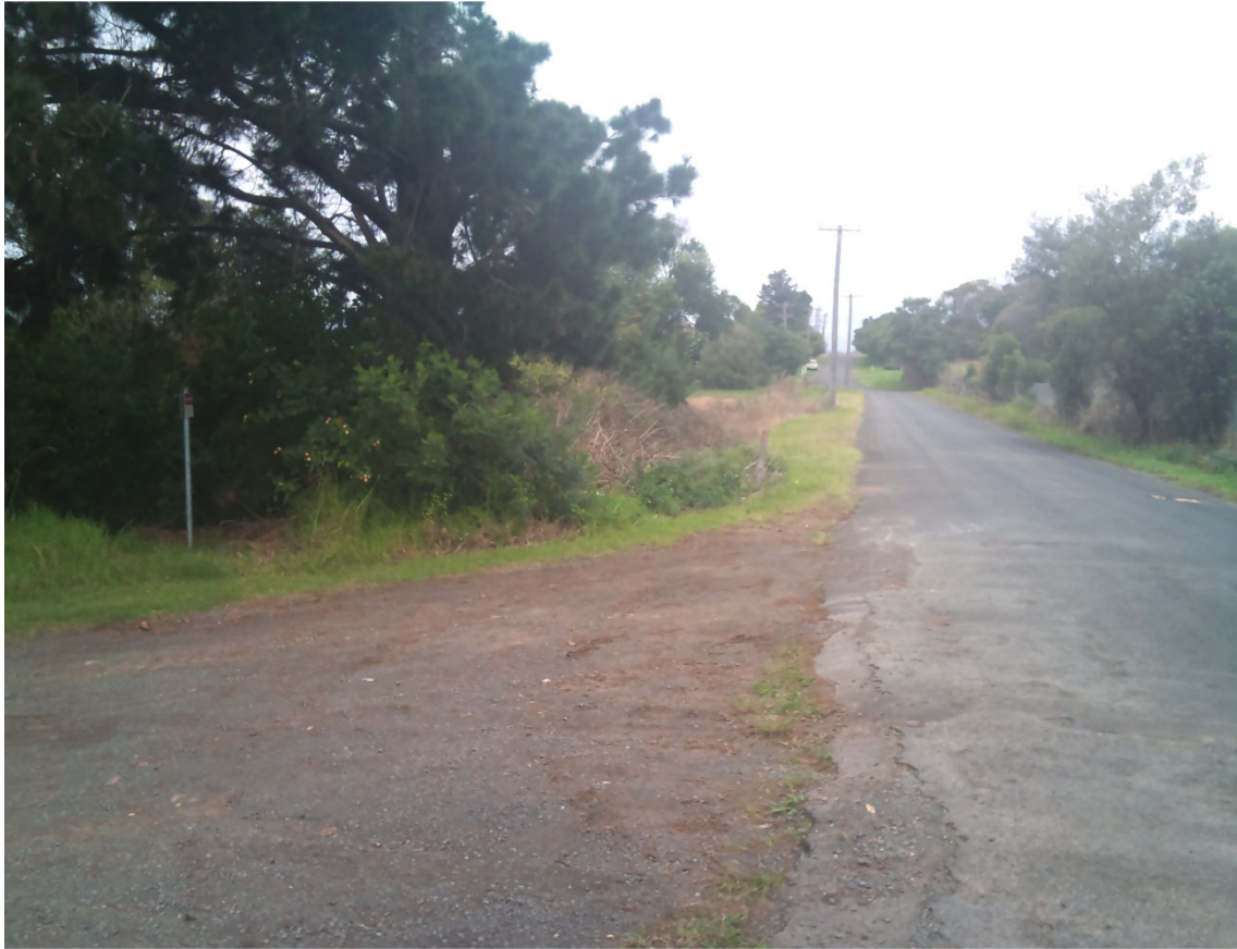
Photo 44- Beginning of sealed section of Railway Street
