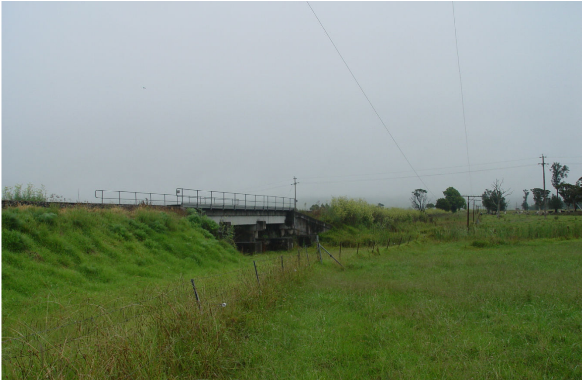
Figure 22: Looking north toward culvert/ bridge #3 and proposed waterway crossing 3 at Abernethys Creek
