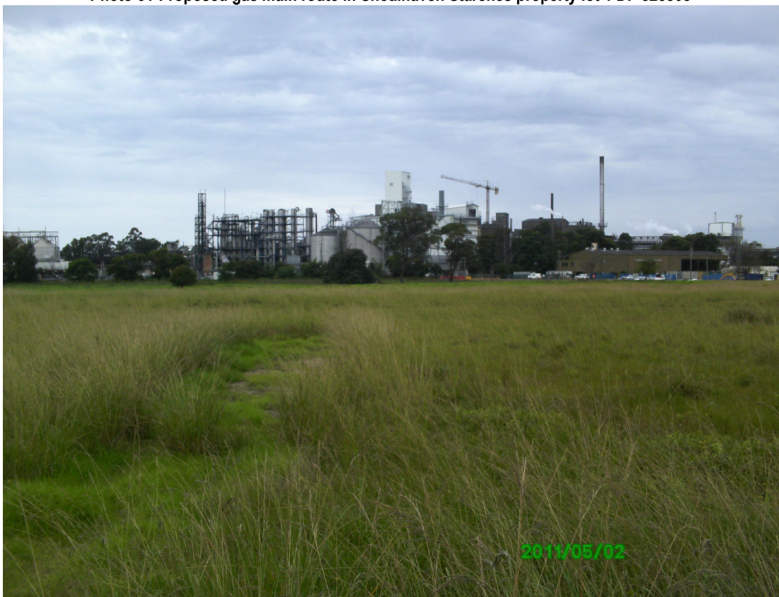
Photo 62- Looking toward Shoalhaven Starches Factory (Manildra), along existing sewer rising main alignment
