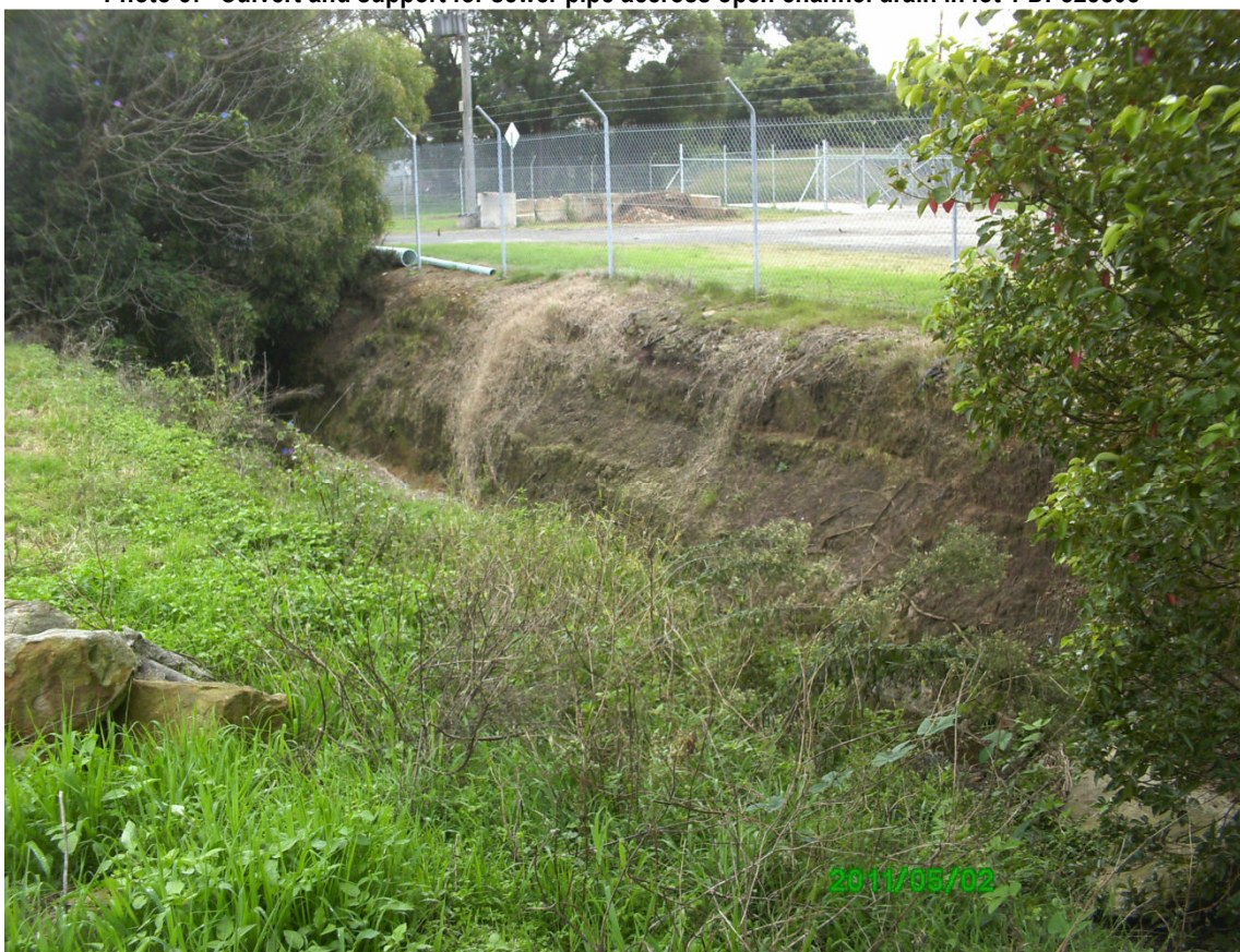
Photo 58-Open channel drain in Lot 1 DP 825808
