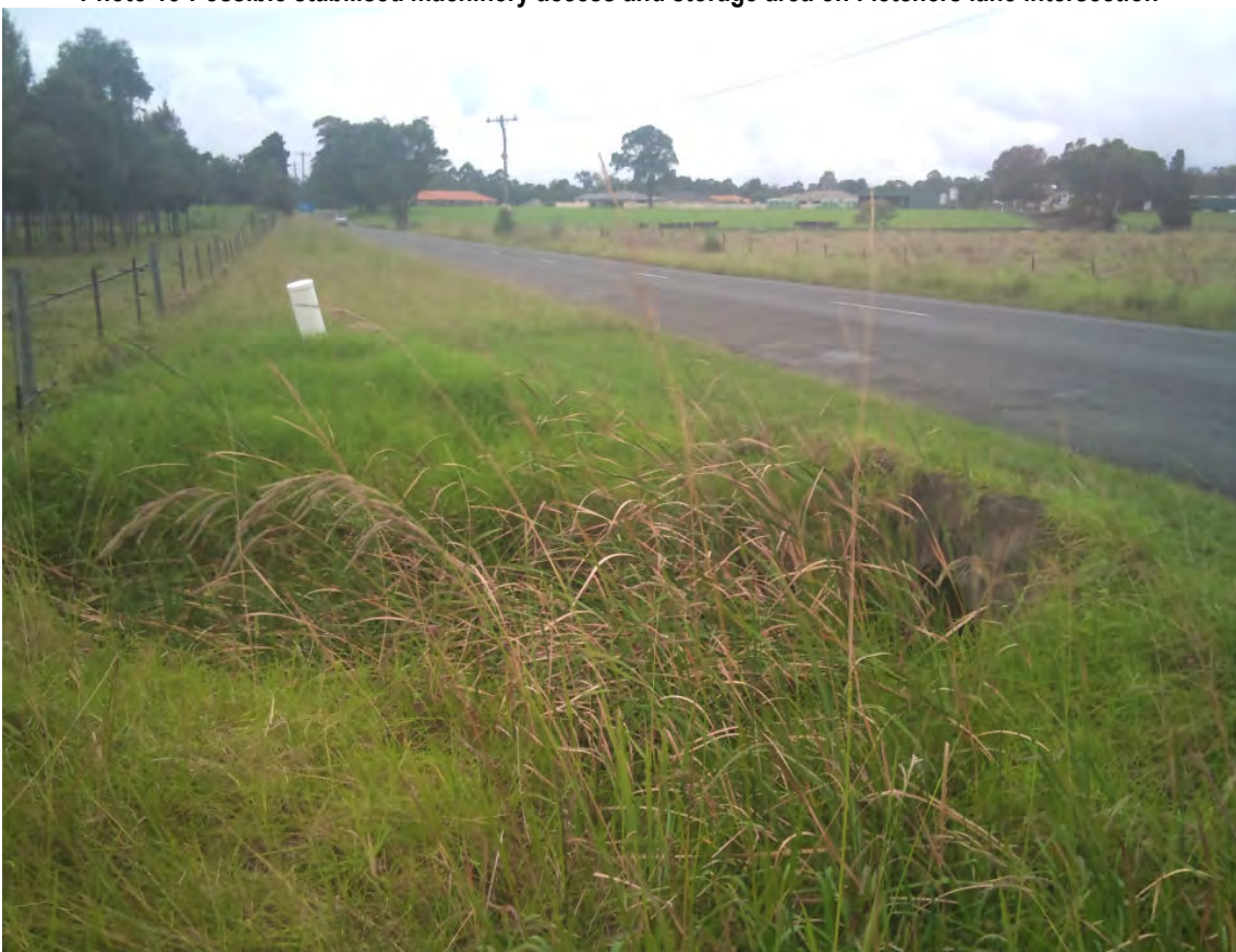
Photo 16- Culvert Headwall and drain leading in Paddock
