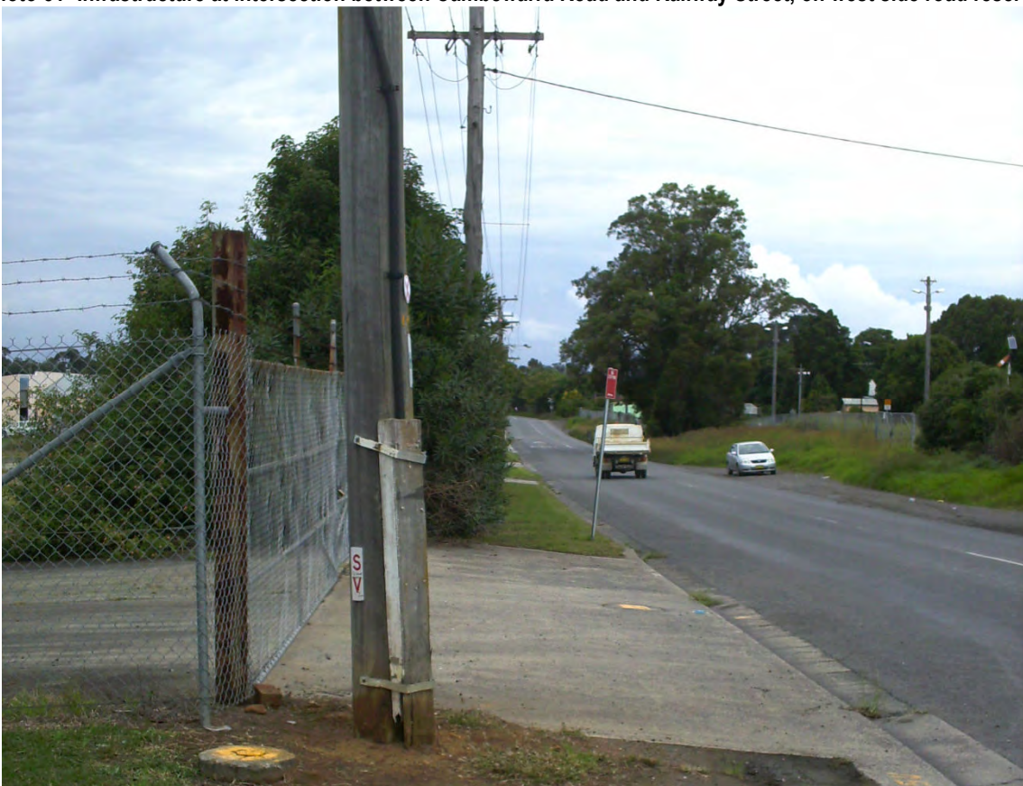
Photo 52- Example of Railway Street Infrastructure in west side of road reserve
