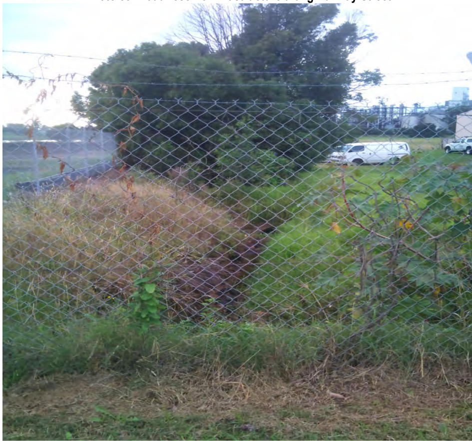
Photo 54- Open channel drain through lot 1 DP825808 at proposed gas main direction change in Railway Street
