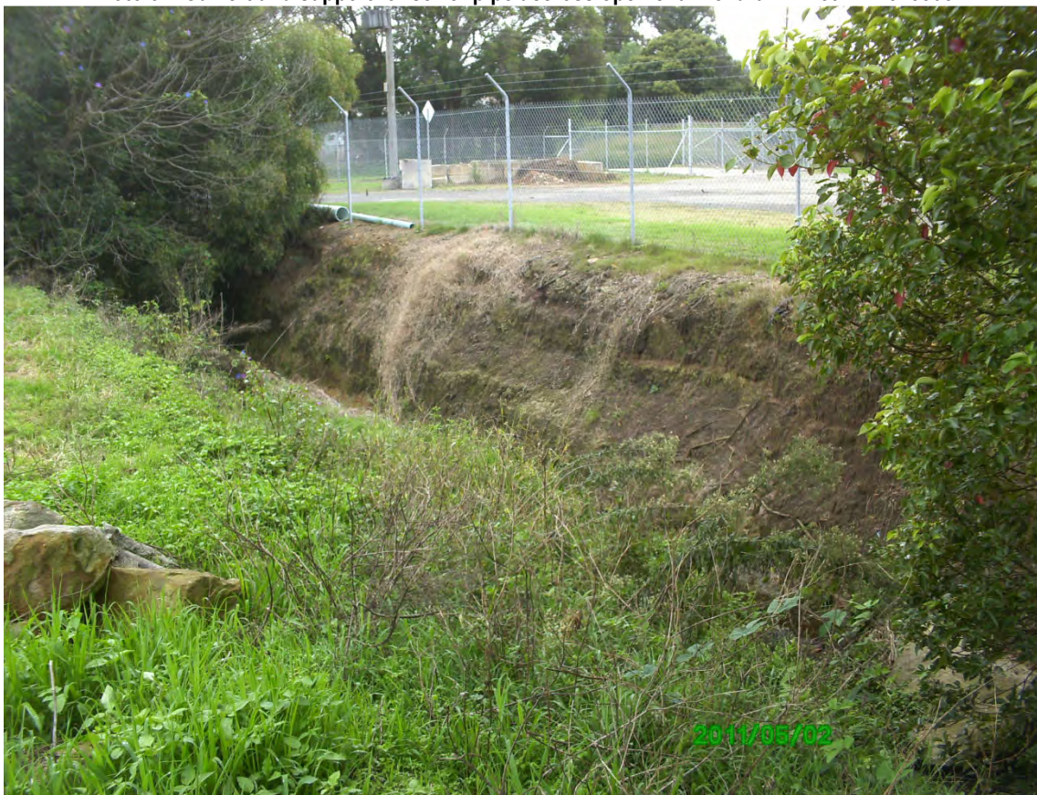
Photo 58-Open channel drain in Lot 1 DP 825808
