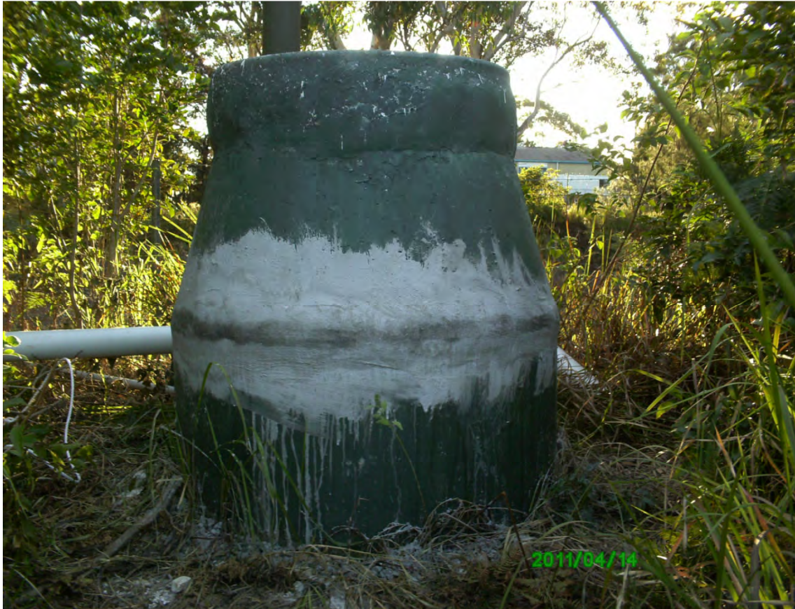
Photo 41-Sewer rising main manhole and vent pipe
