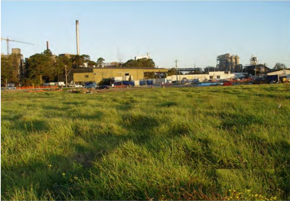
Photo 63- Proposed gas main route through Shoalhaven Starches paddock, looking toward interim packing plant
