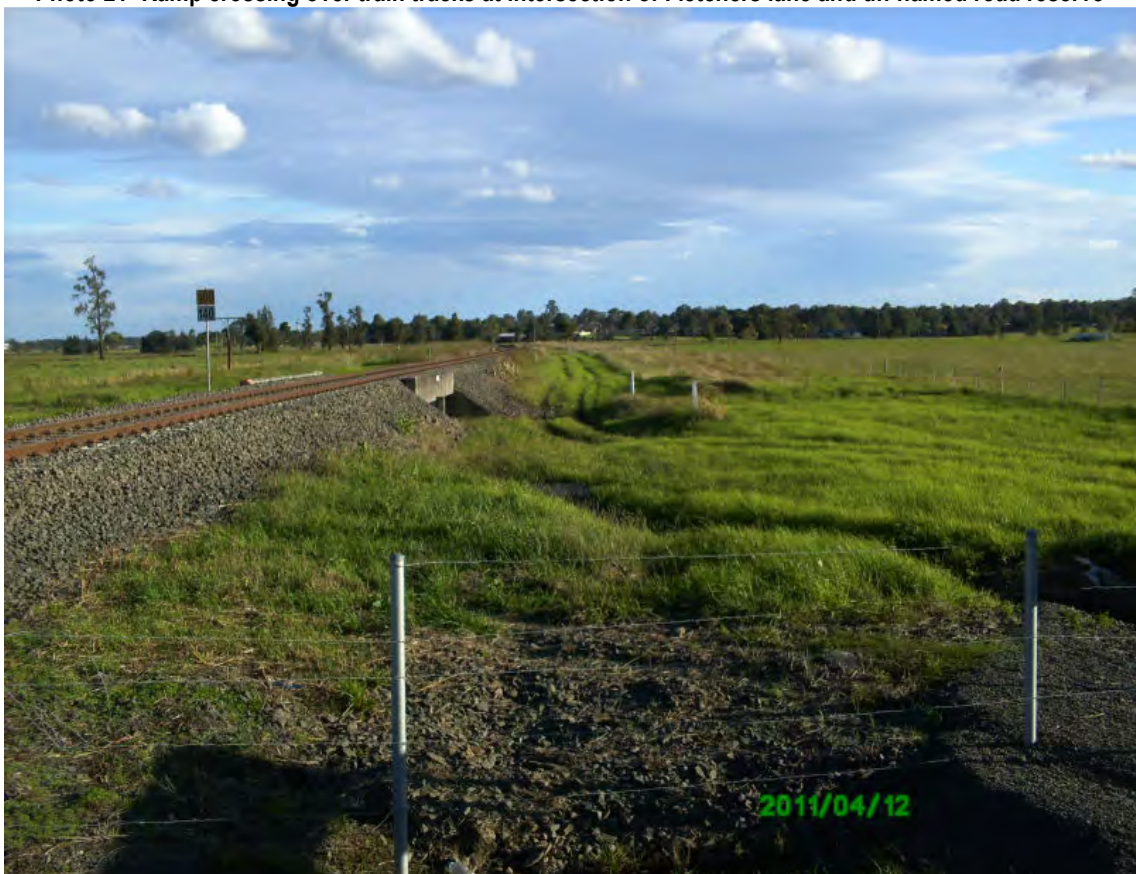
Photo 22-Large culvert in Railcorp railway reserve
