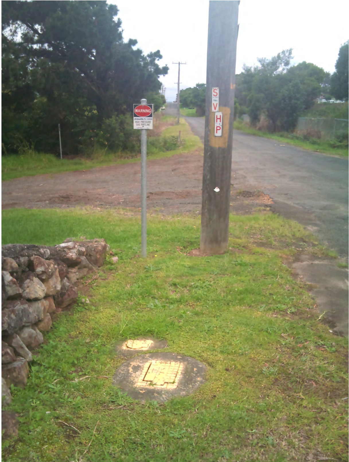
Photo 43-Water main, power pole and existing gas main infrastructure in Railway Street
