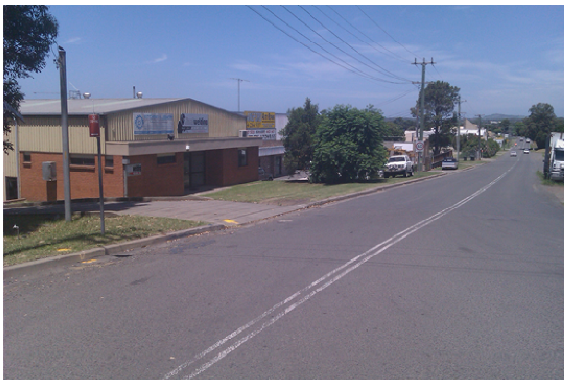
PHOTOGRAPH 2-9 PIPELINE ROUTE LOOKING SOUTH DOWN RAILWAY STREET
