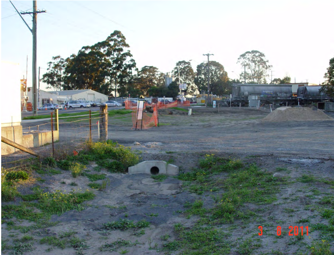
Photo 65- Civil works at most likely position of proposed gas main crossing of Bolong Road
