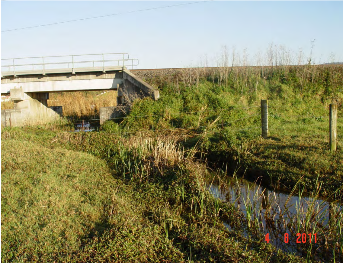
Photo 27- Large railway bridge at second proposed waterway crossing
