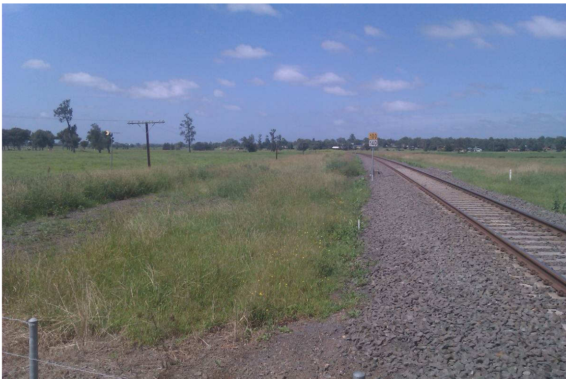
PHOTOGRAPH 2-5 PIPELINE ROUTE ALONG SOUTH COAST RAILWAY (LOOKING SOUTH)
