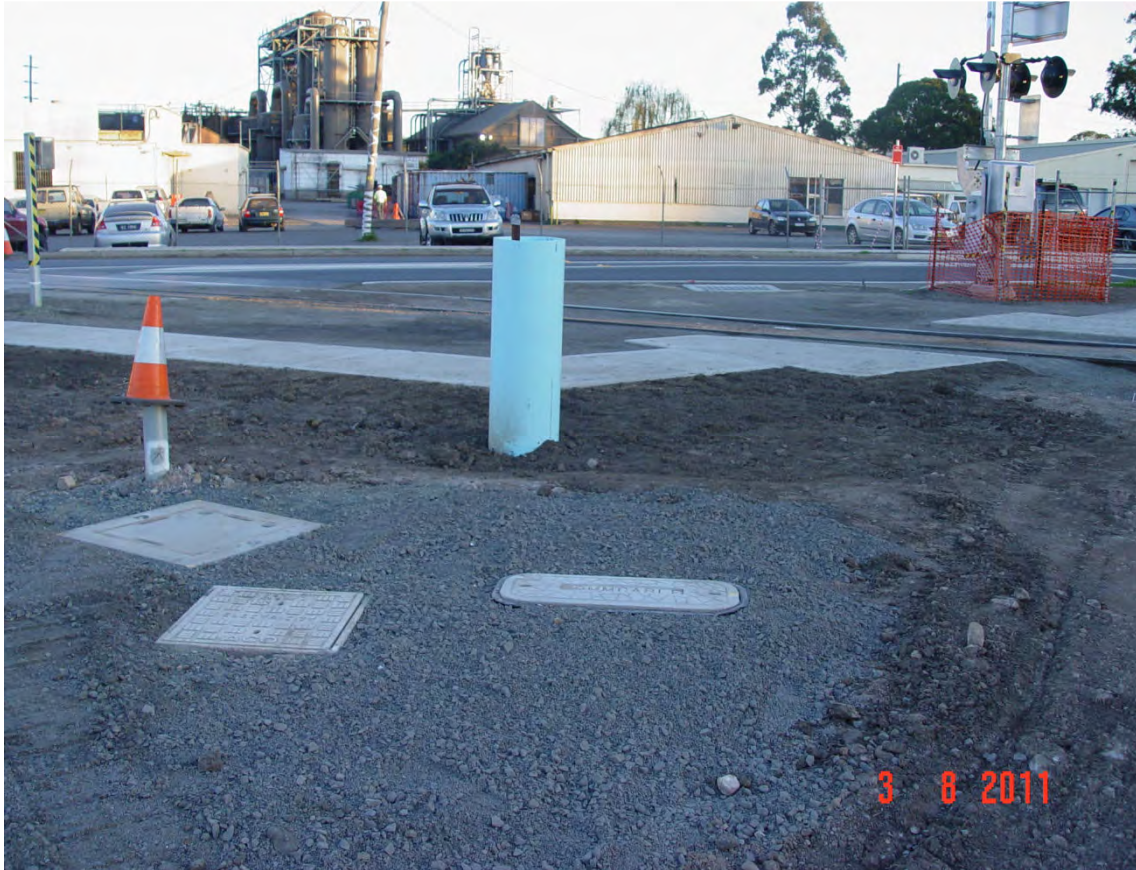
Photo 67-Bolong Road showing infrastructure in vicinity of proposed gas main crossing
