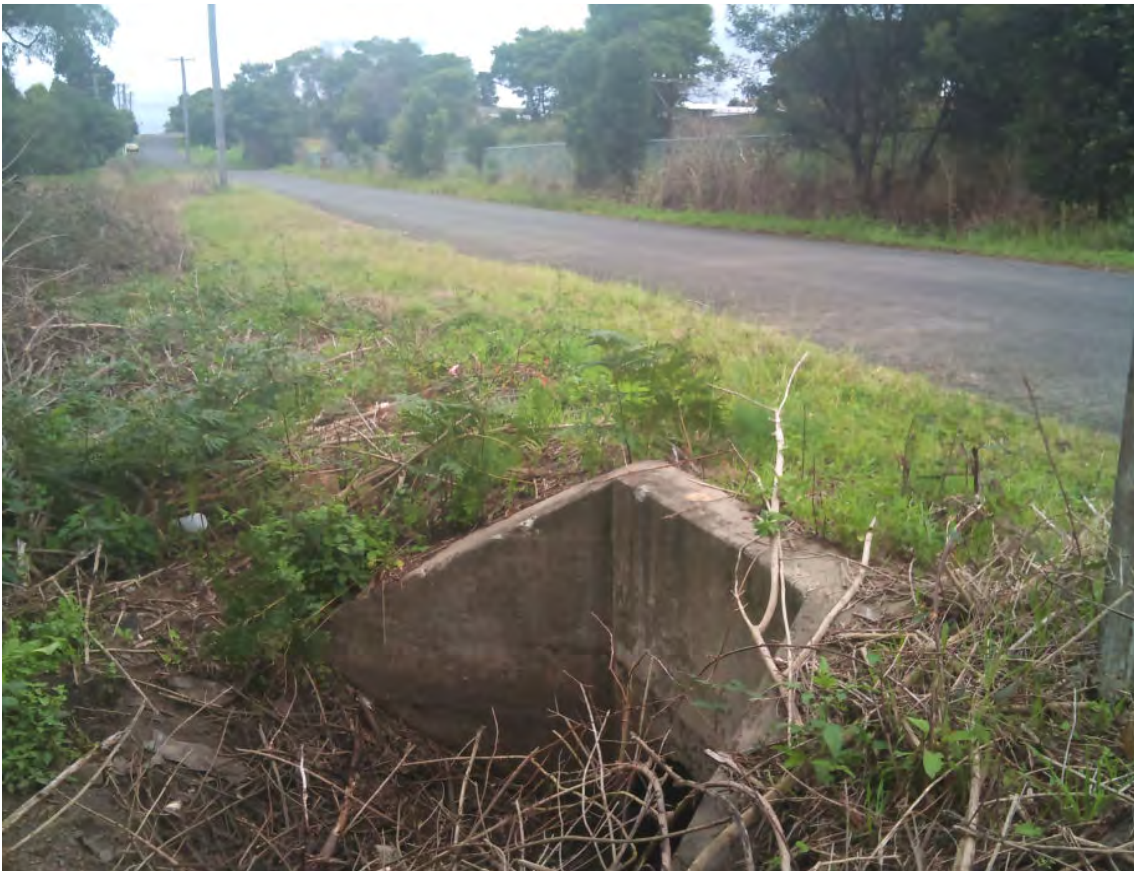
Photo 45- Stormwater headwall and culvert in Railway Street
