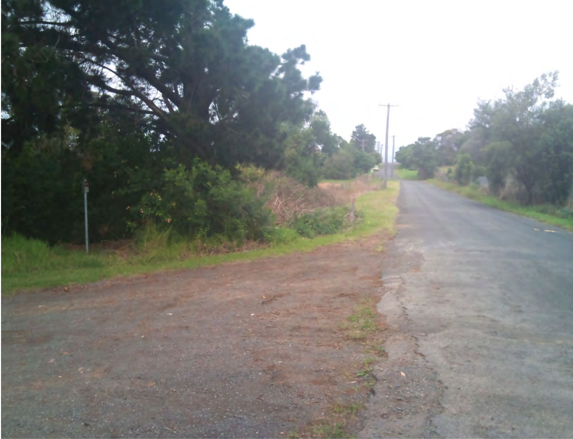
Photo 44- Beginning of sealed section of Railway Street
