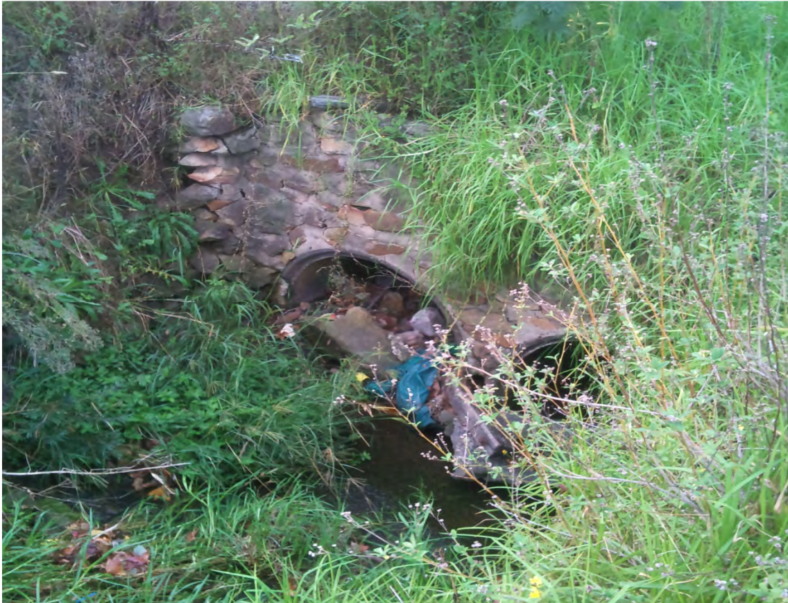
Photo 57- Culvert and support for sewer pipe accross open channel drain in lot 1 DP825808
