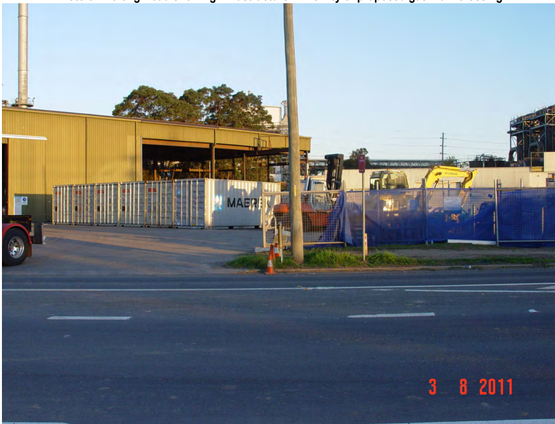
Photo 68- Shoalhaven Starches interim packing plant on south side of Bolong Road
