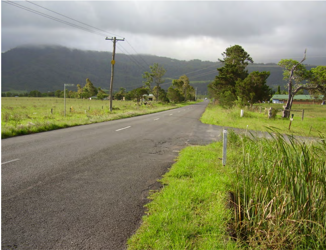
Photo 13- Culvert headwall (bottom right) on Meroo Road and Fletchers lane intersection
