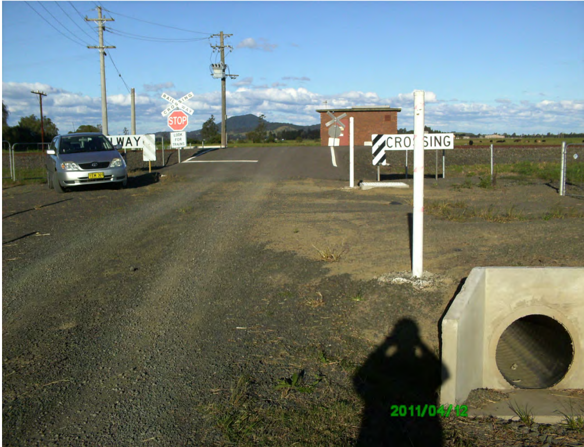
Photo 21- Ramp crossing over train tracks at intersection of Fletchers lane and un-named road reserve
