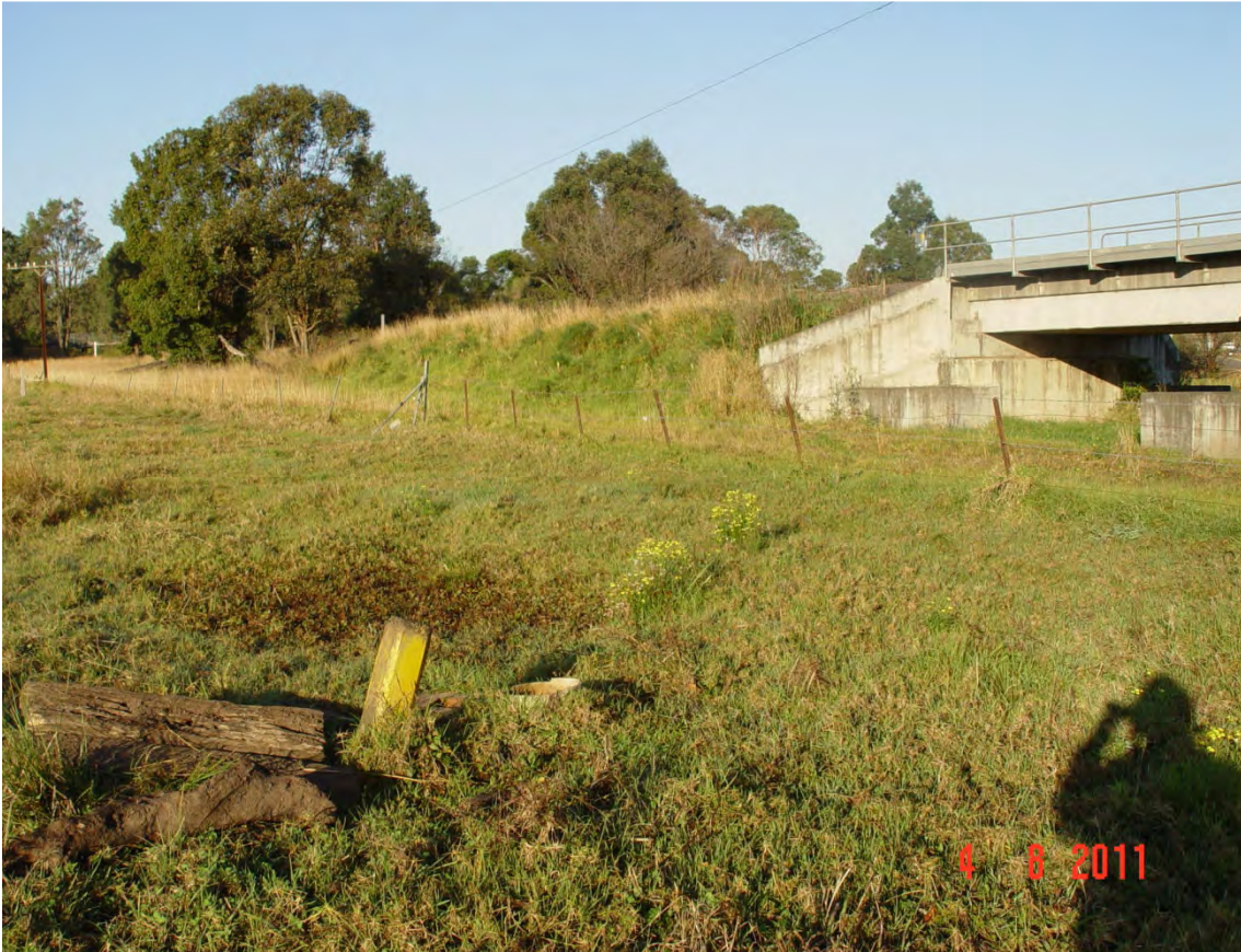
Photo 25-Scour valve in un-named road reserve adjacent to second proposed waterway crossing, south of Edwards Avenue
